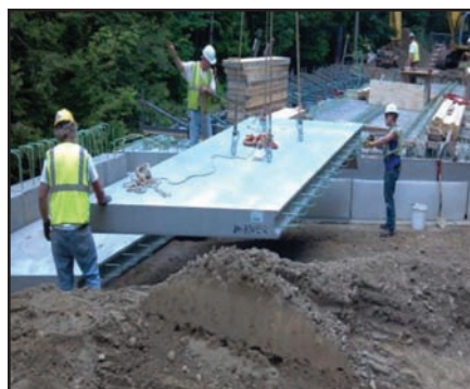
Setting approach slabs
