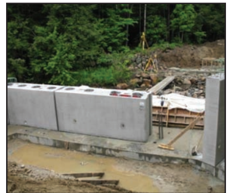
Setting abutment pieces
