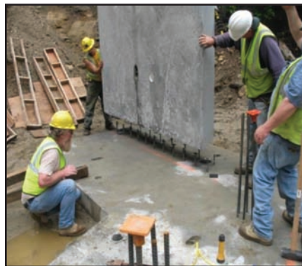
Setting first wingwall
