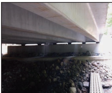
Next Beams installed on bearing pads
