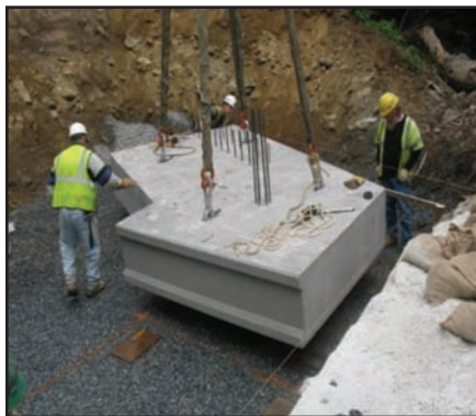
Setting first footing piece
