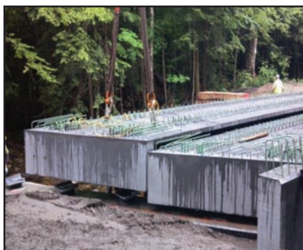
Setting NEXT 32F beams
