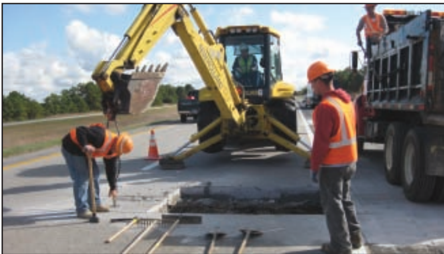
Saw Cut and Remove Slabs To Be Replaced
