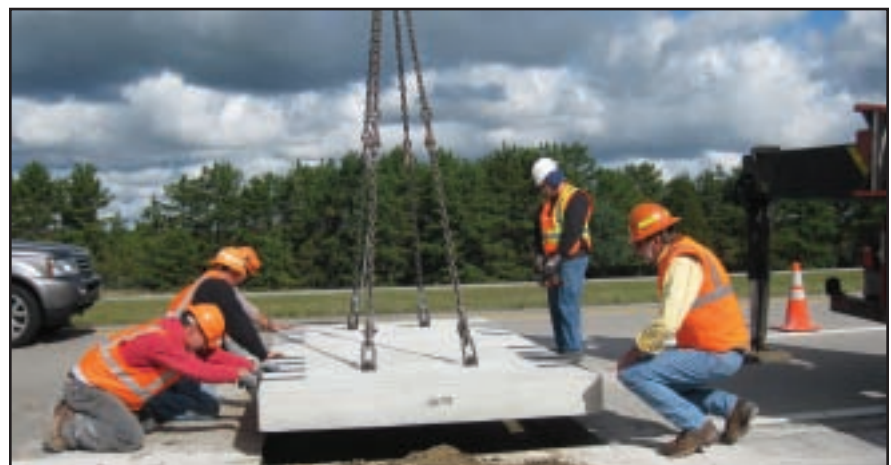
Set New Precast Road Slabs
