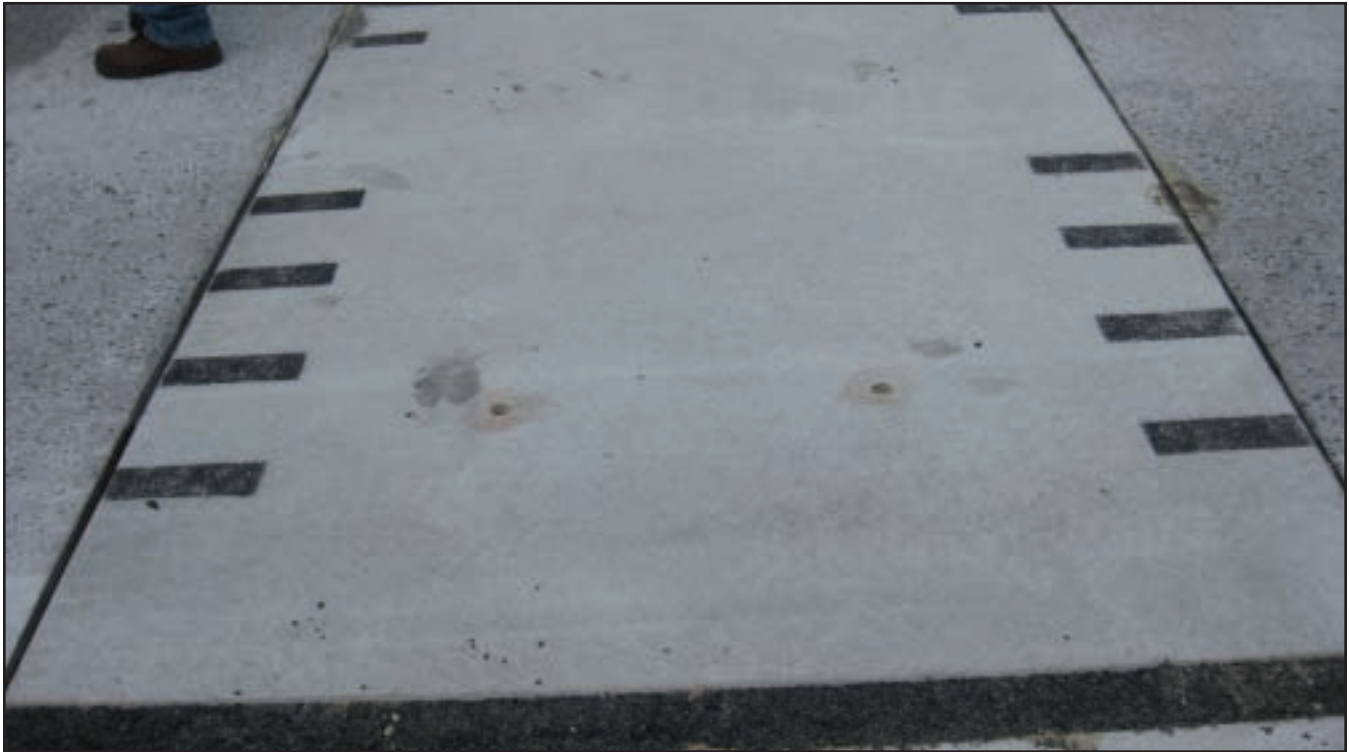
Finished Roman Road System replacement segment
