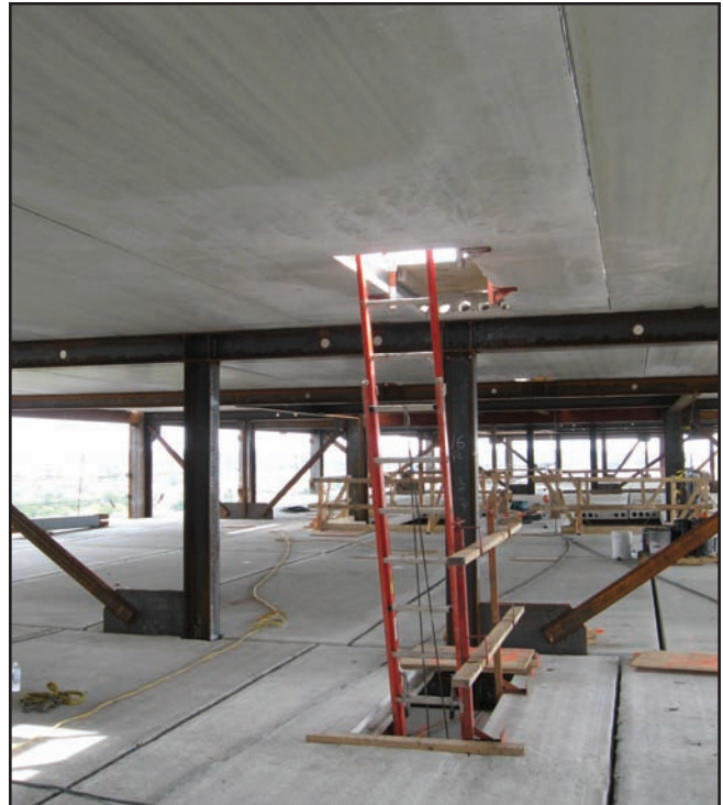
Mechanical openings thru plank, staggered truss support
