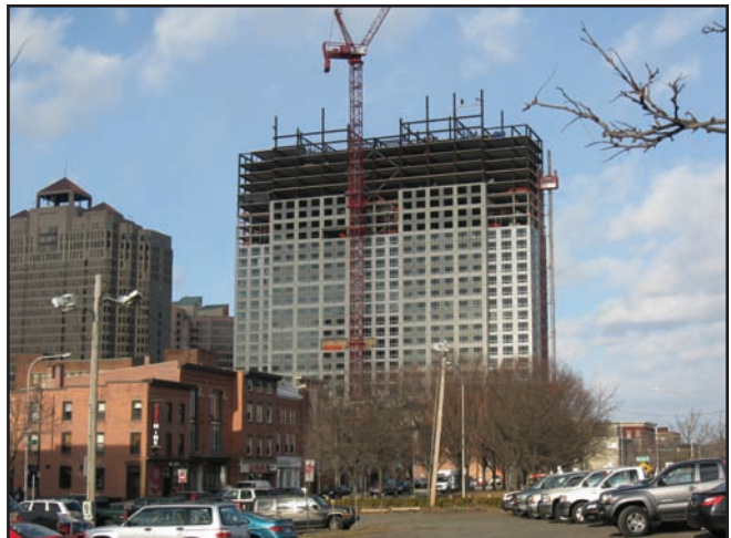
Plank partially erected on level 30, precast wall panels close behind
