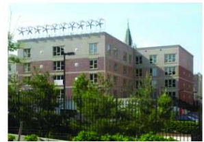
[10] 1 kW low speed wind turbines mounted on precast parapets help generate up to 90% of the building's electrical needs during the evenings.
