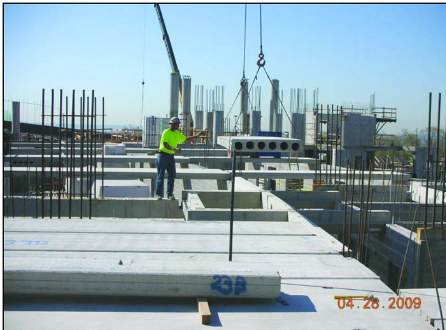
2 Hr. Fire Rated Hollow-core plank installation on curved building footprint
