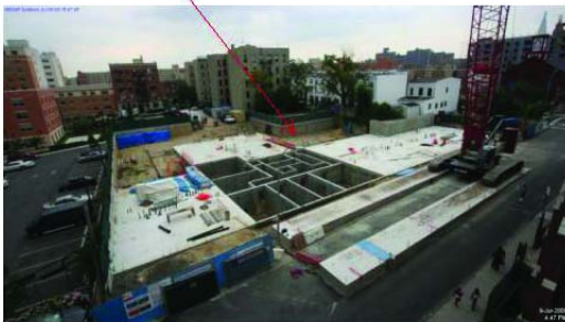
Urban sites with very limited space for construction
