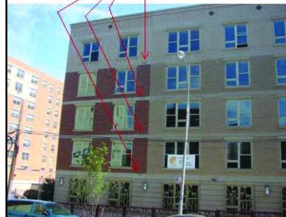
Exterior vent thru plank hollow cores saved duct work & reduces energy use
