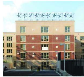
[10] 1 kW low speed wind turbines mounted on precast parapets help generate up to 90% of the building's electrical needs during the evenings.
