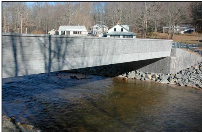
Completed Structure, Downstream Elevation
