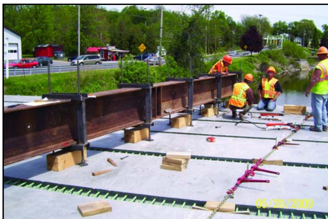
Jacking frame used to adjust beam cambers
