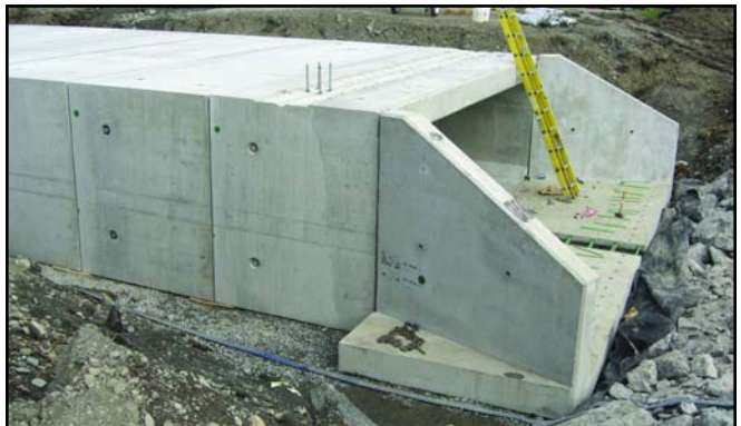
Then Place 7 Box Culvert Sections, and Repeat...
