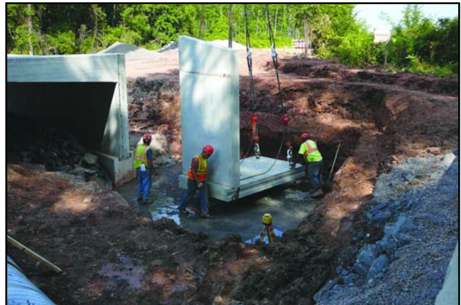
Setting Precast Wingwall
