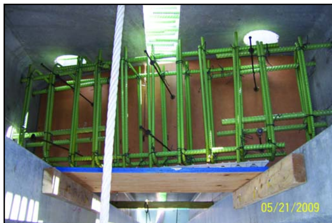
Forming and reinforcing for lateral diaphragm
