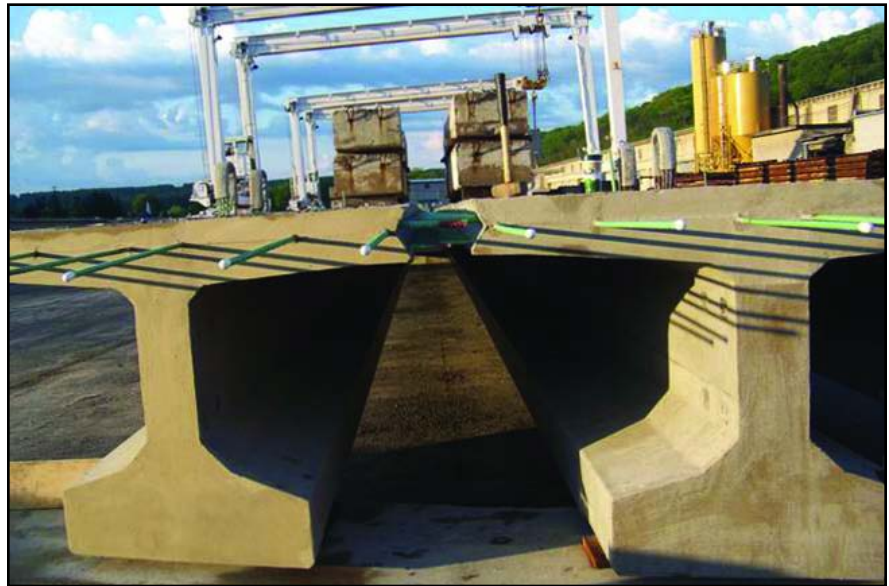
Decked bulb tee beams being set up in Northeast Prestressed Products plant Photo provided by Northeast Concrete Products
