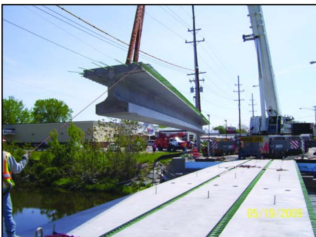
Beams being erected onsite
