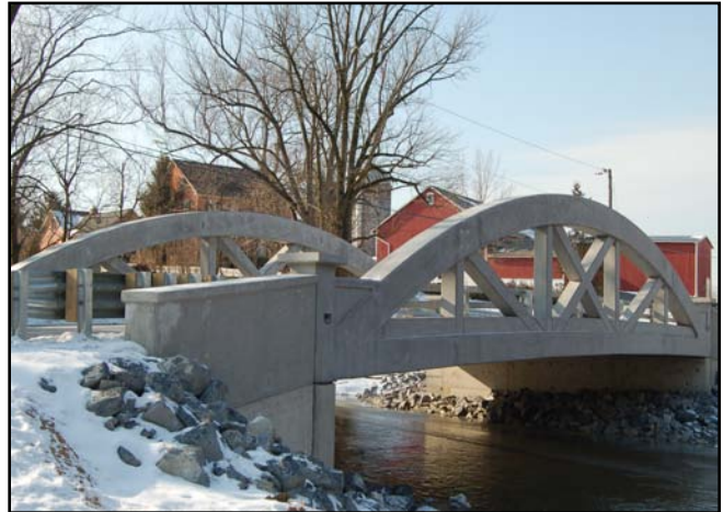
Auction Road Bridge (December, 2008)
