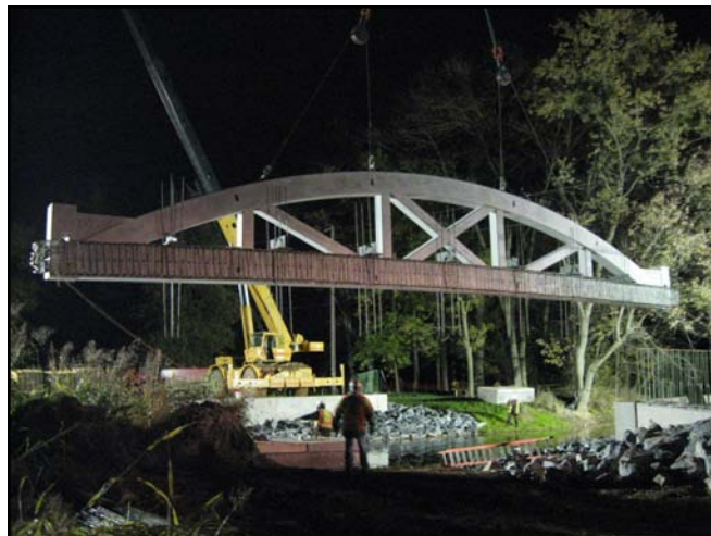
Overnight Arch Erection
