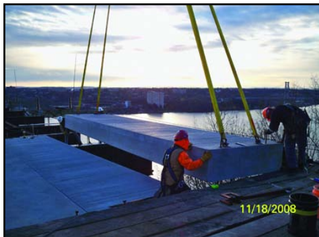
Installation of precast deck units
