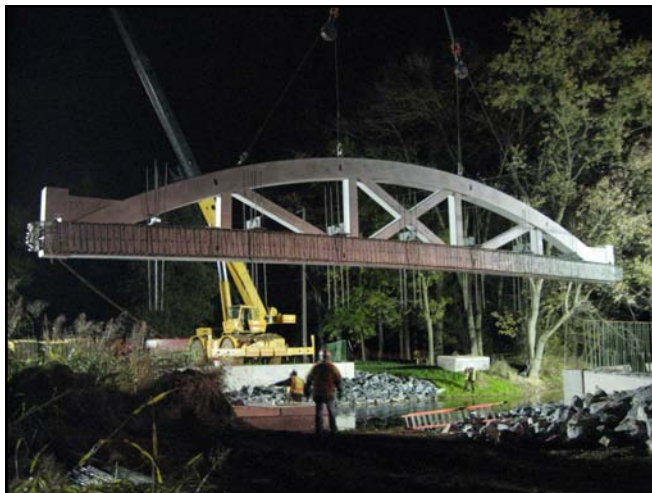
Overnight Arch Erection
