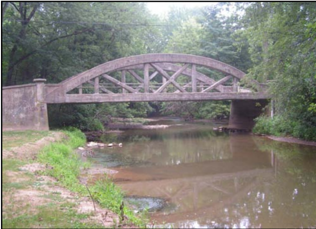
Original Auction Road Bridge
