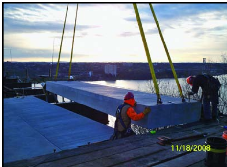
Installation of precast deck units
