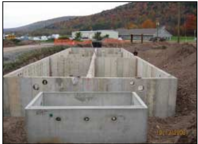
Septic tank & sand filter dosing valve vault, before covers placed
