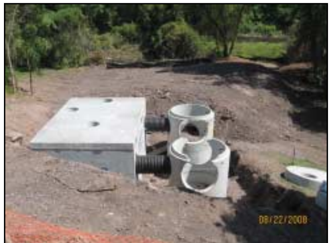
Bypass manholes being connected to the Vortech unit
