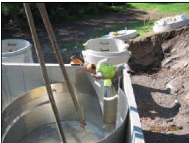
Checking for level the hard way
