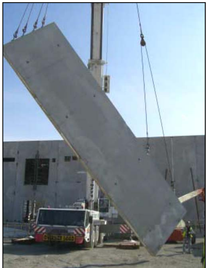
Precast insulated panel being lifted for placement.
