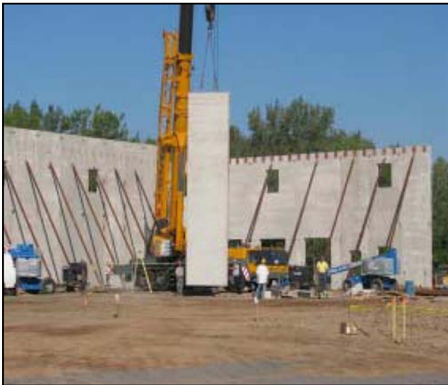
Insulated bearing panel erection
