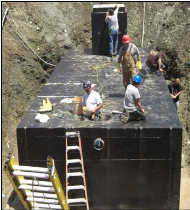
13,000 Gallon Kon-Seal-Kon-Lock Watertight Gasketed Septic Tank©
