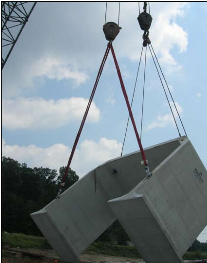
Each precast arch has an 18’ internal span, 12’ internal rise, and is 8’ long, cast with monolithic foundation pads
