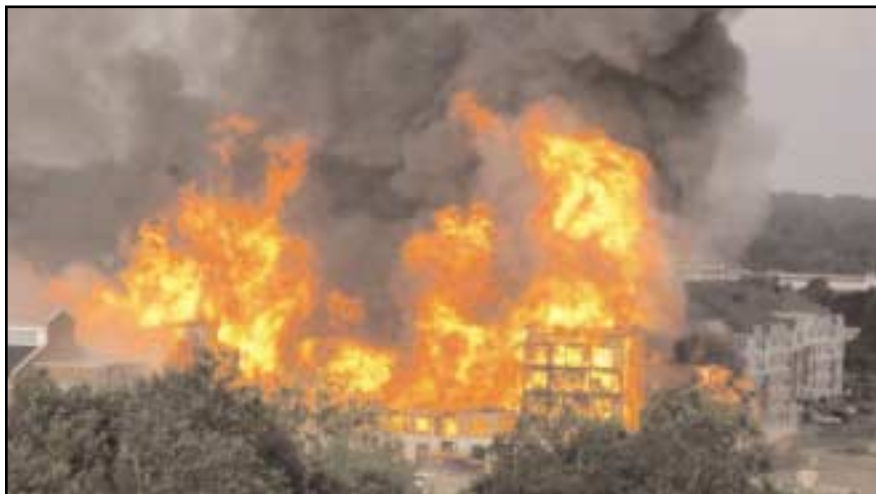
Conshohocken, PA – 8 Alarm Blaze Destroys 185 Apartments
