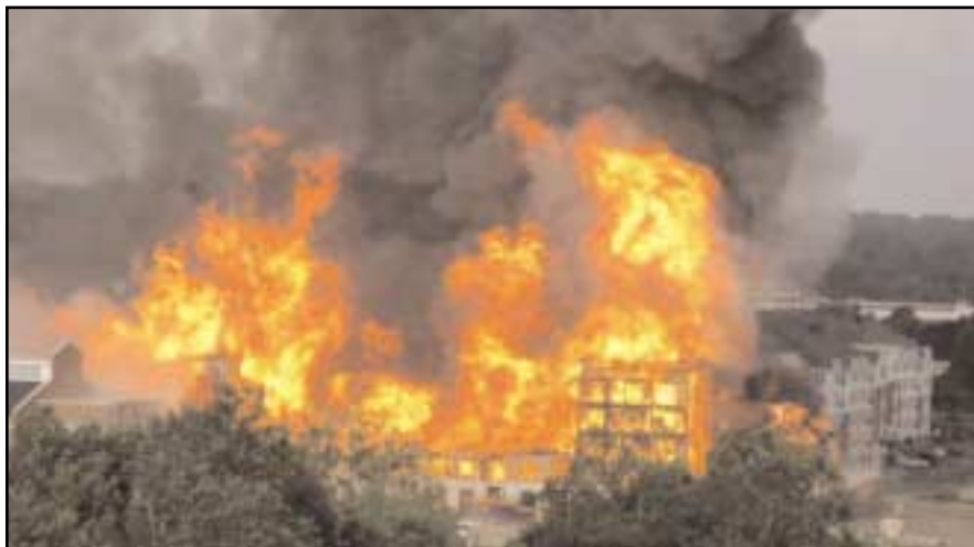
Conshohocken, PA – 8 Alarm Blaze Destroys 185 Apartments
