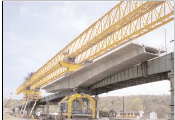
Roslyn Viaduct, Roslyn, NY Photo by NYSDOT
