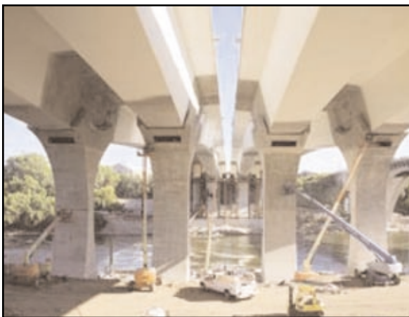
Curving piers supporting each box girder ensures redundancy of new I-35W bridge.
