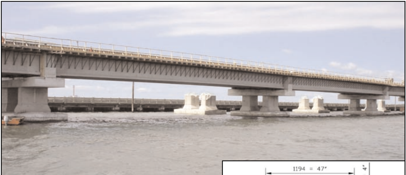
Rt. 52 Causeway, Somers Point, NJ Photo by Bayshore Concrete Products Corp.
