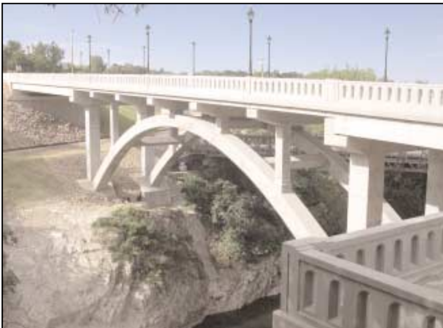
Lime Kiln Bridge, Burlington, VT today
