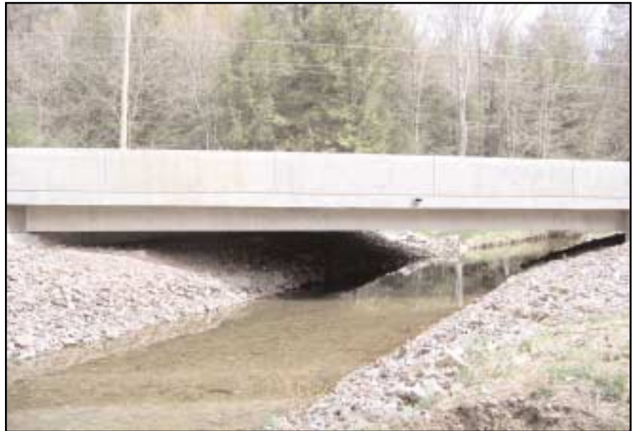
PA Luzerne Co., SR 118 (GC: Susquehanna Supply) Six 48” wide by 27” deep by 60’ long Spread Box Beams (24 tons each)
