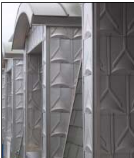
Closeup of Silverleaf Hall mansard construction and exterior detailing.
