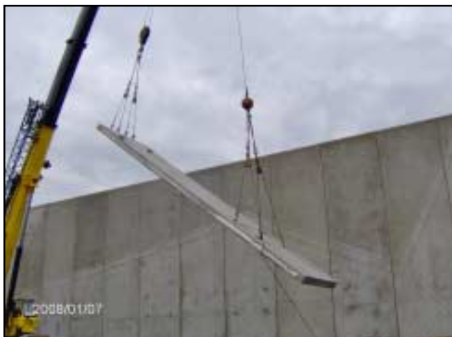
Ten foot wide panel being swung into position.
