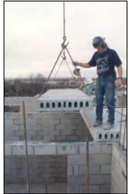
Typical plank erection, WSAAF Barracks, Fort Drum.
