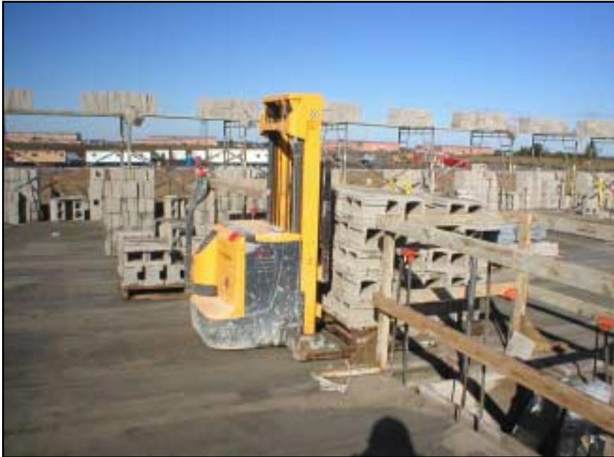
Not typical plank loading, Hampton Inn, Warwick.
