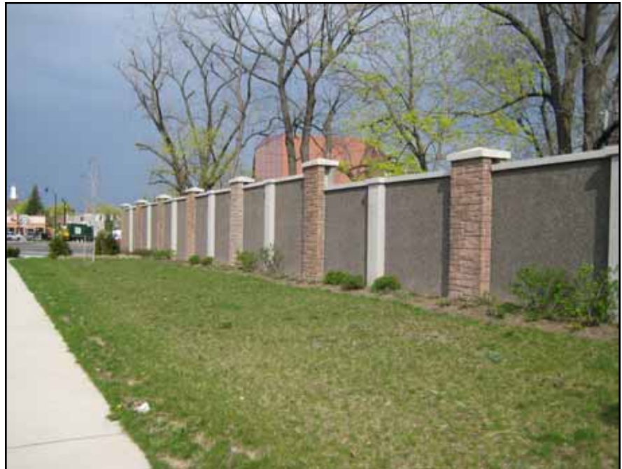
New West Ridge Road Sound Walls
