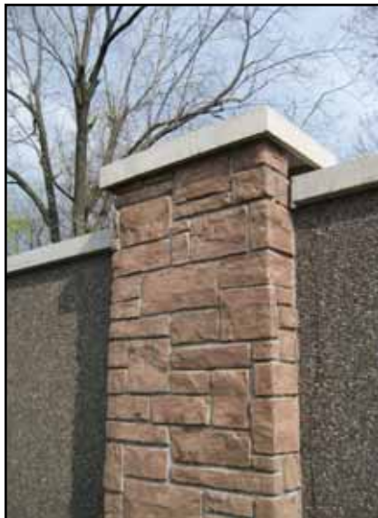
Columns Feature Ashlar Stone Finish
