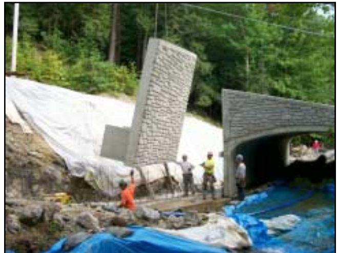
Precast wingwall installation
