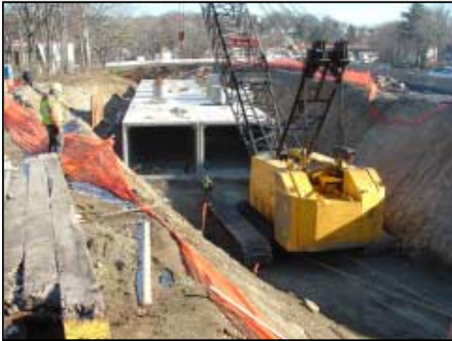
Relocate Crane for Last 8 pcs
