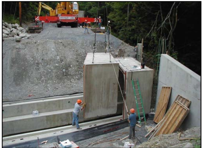
Installation of Rigid Frame Units
