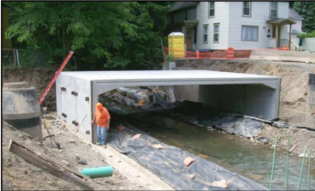
Installation of 29'-9" Span Units over Steele Creek
