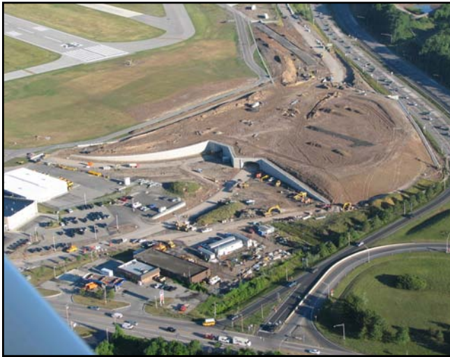
Tunnels Relocate Roadways Underground at End of Runway
