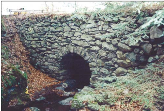
Original Laid-up Stone Arch at Upstream Face
