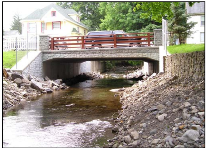
Replacement Third St. Bridge over Steele Creek, Herkimer County
