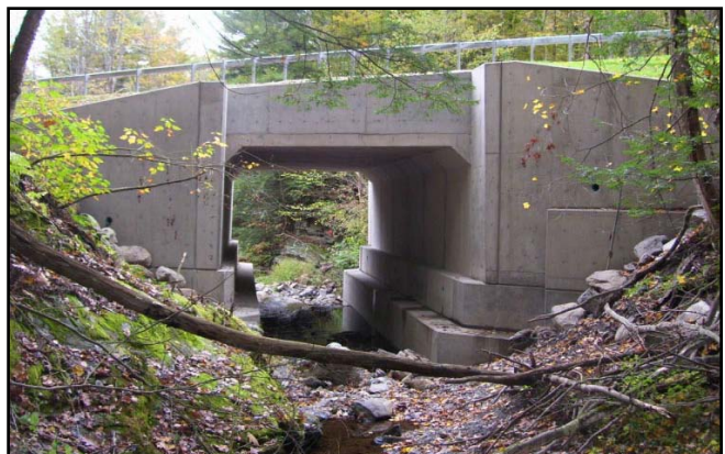
Completed Structure — Precast Three-Sided Culvert on Stepped Concrete Footings
