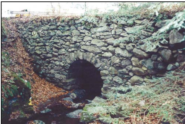
Original Laid-up Stone Arch at Upstream Face
