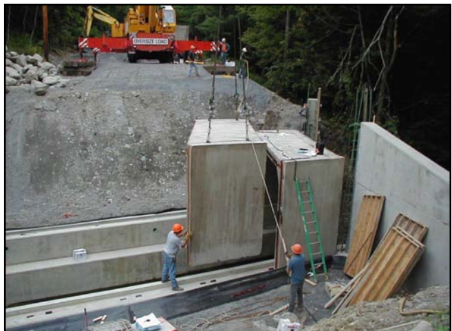
Installation of Rigid Frame Units
