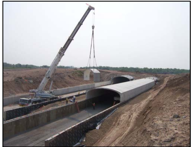
Installation of Twin Tunnels Using Precast Arch Members
