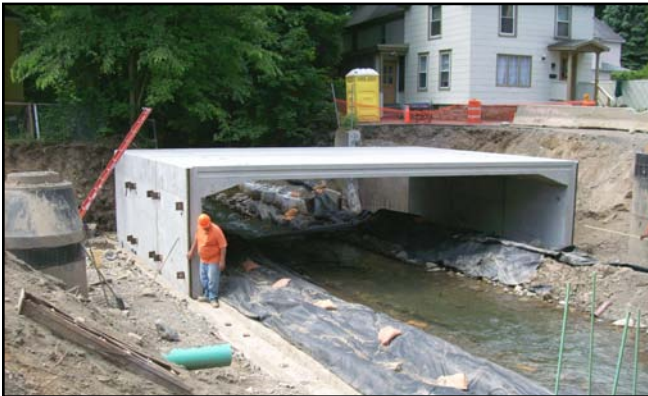
Installation of 29'-9" Span Units over Steele Creek
