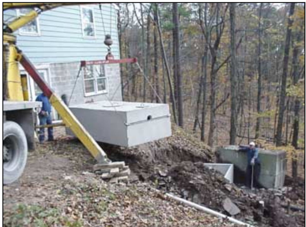
Septic tank being installed at an Ulster County home site
