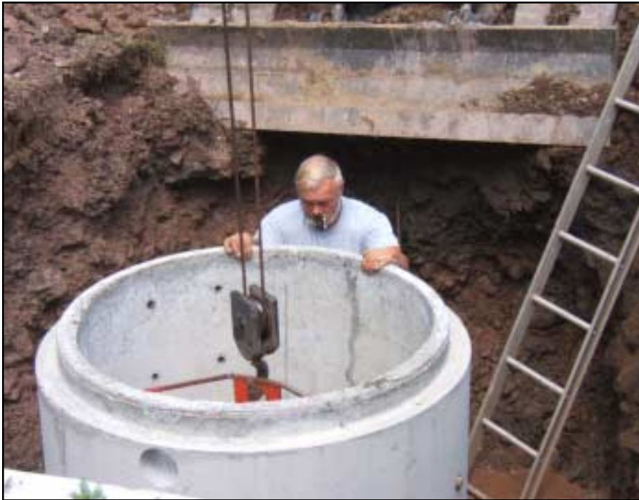
Installation of pump chamber for a septic system in Margaretville
