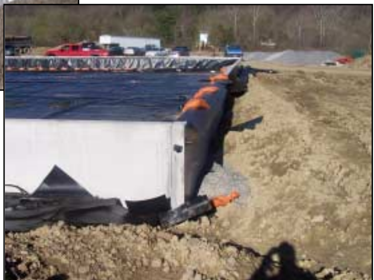
Walls post-tensioned, geomembrane installed
