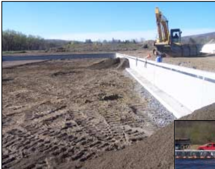
'L' Sections installation
