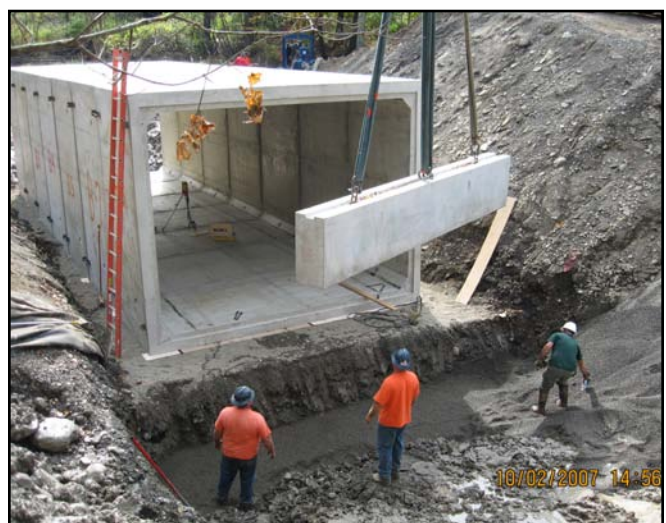
Preparing to set toe-wall
