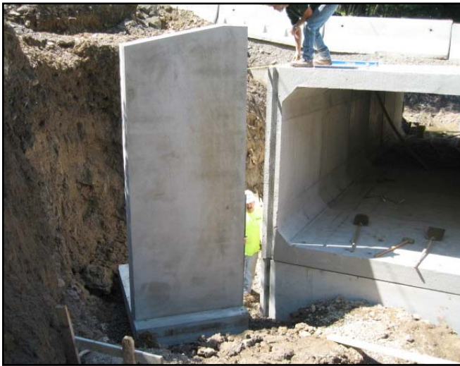
L-shaped wing wall being placed
