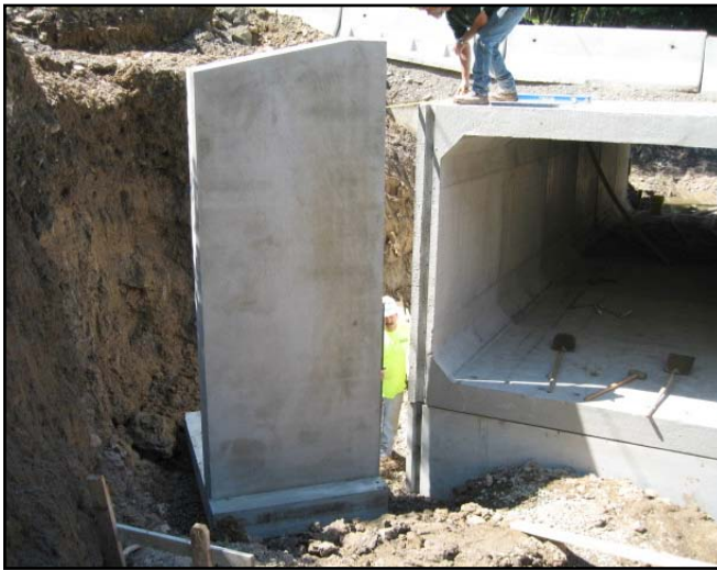
L-shaped wing wall being placed
