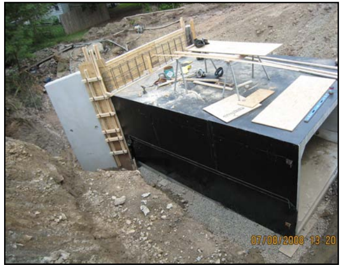
Readying connecting and head-wall pours
