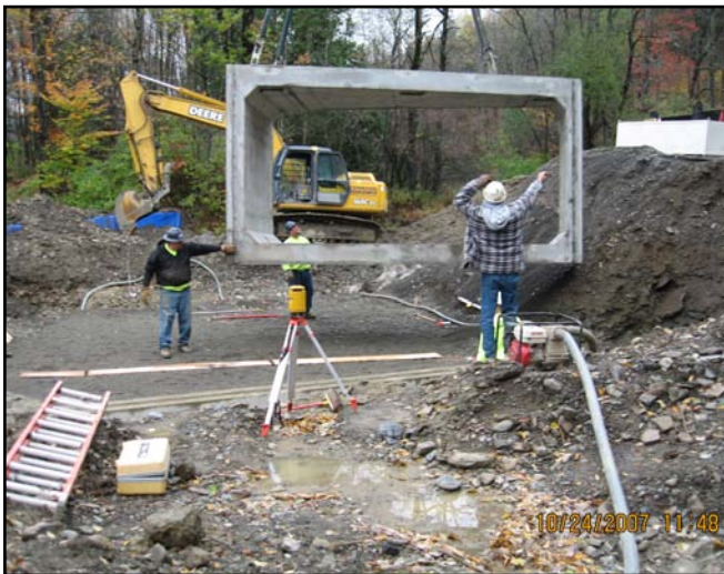
Lower Cross Road, first pieces going in
