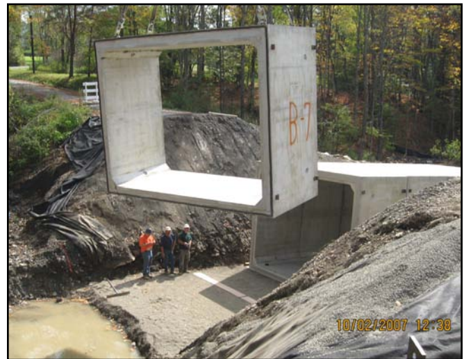
(All photos by Lamont Engineers)
