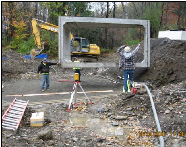
Lower Cross Road, first pieces going in
