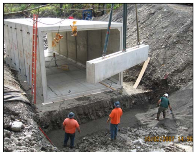
Preparing to set toe-wall
