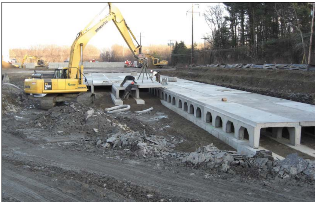
Fast Winter Installation of Storm Water Detention System
