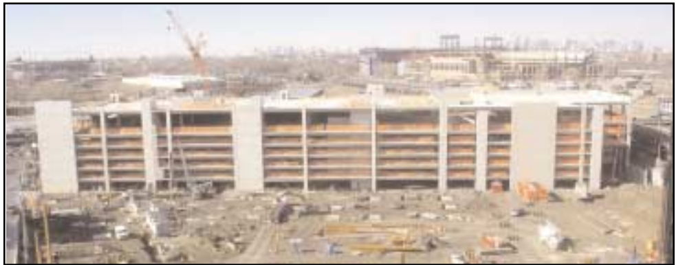
Sky View Parc garage construction nearing completion
