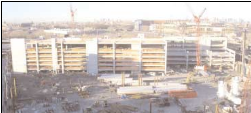
Sky View Park, Flushing, taking shape
