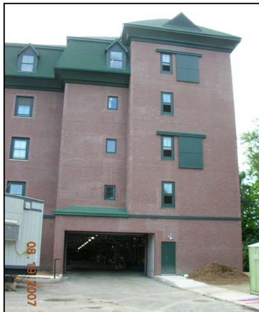
Entrance to first level parking areas
