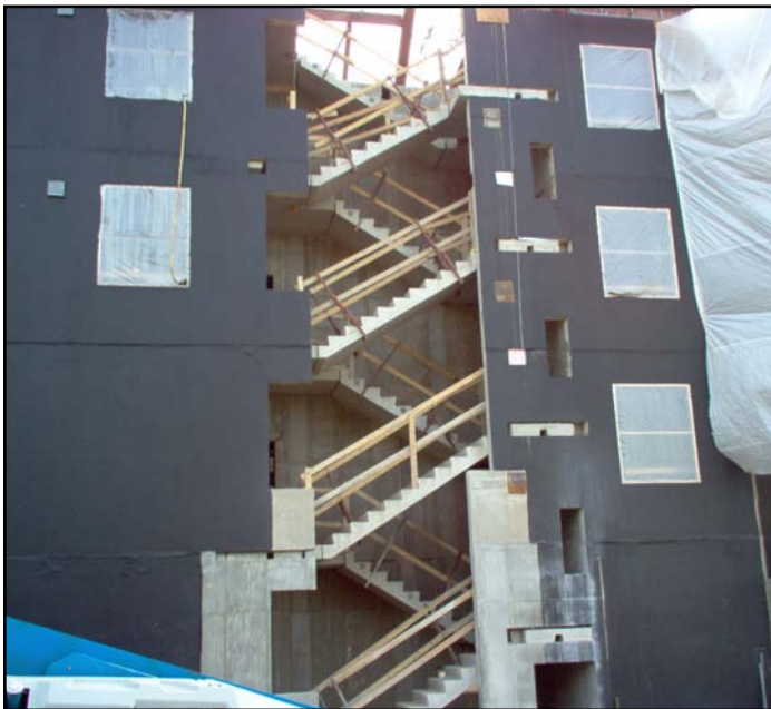
Using precast stairs and landings for safe access
