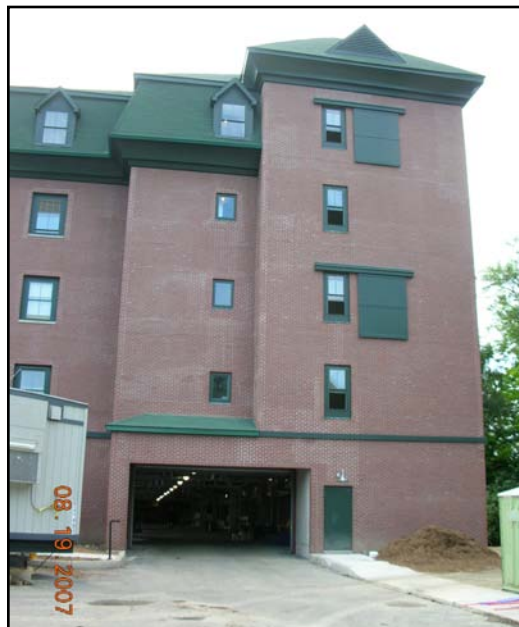
Entrance to first level parking areas
