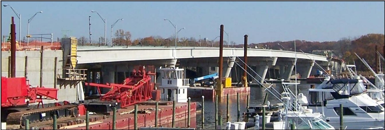
Route 70 Bridge over Manasquan River
