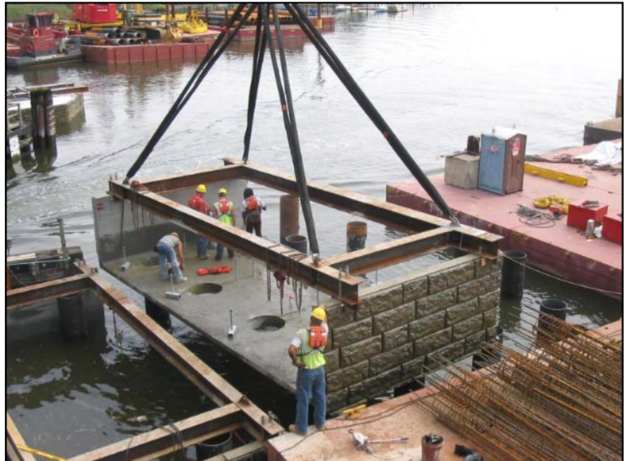
Precast Pier Segment Being Installed
