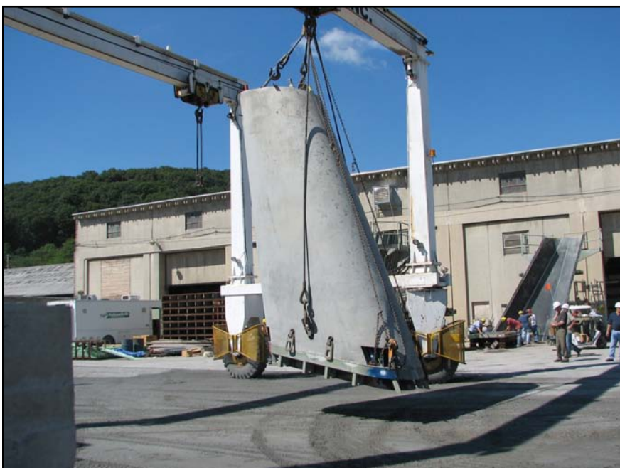
Tapered Precast Columns After Removal from Forms at Precast Plant
