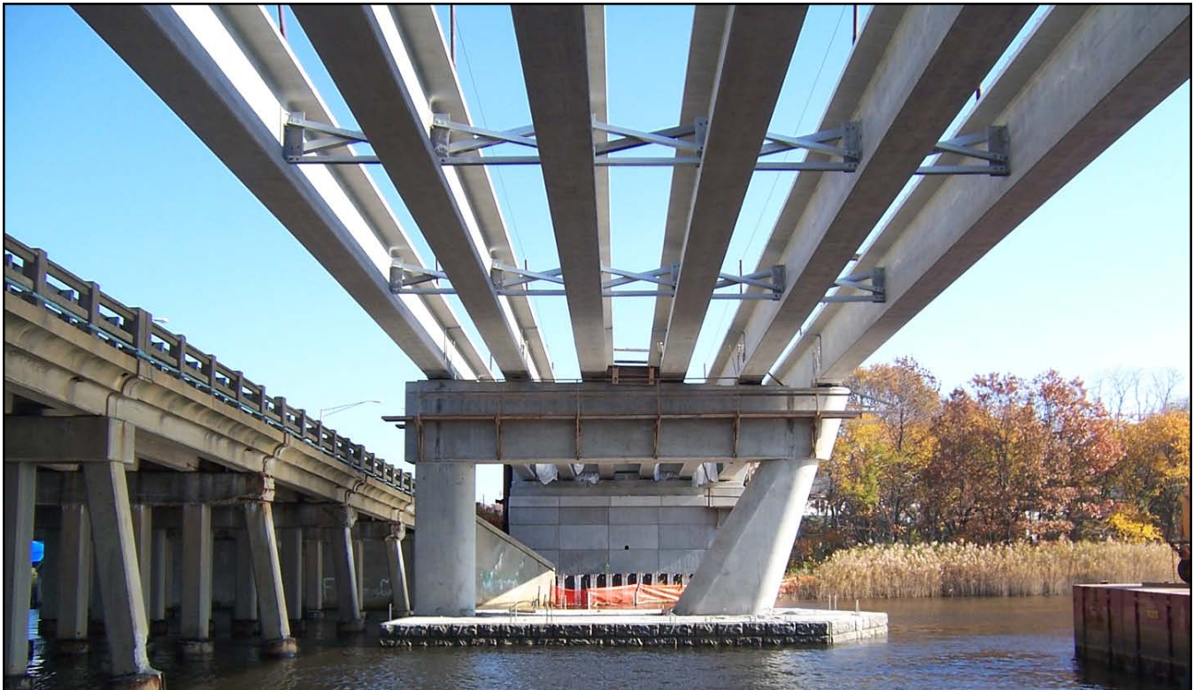
PCEF Bulb Tee Beams, Pier Caps and Columns installed over the Manasquan River
