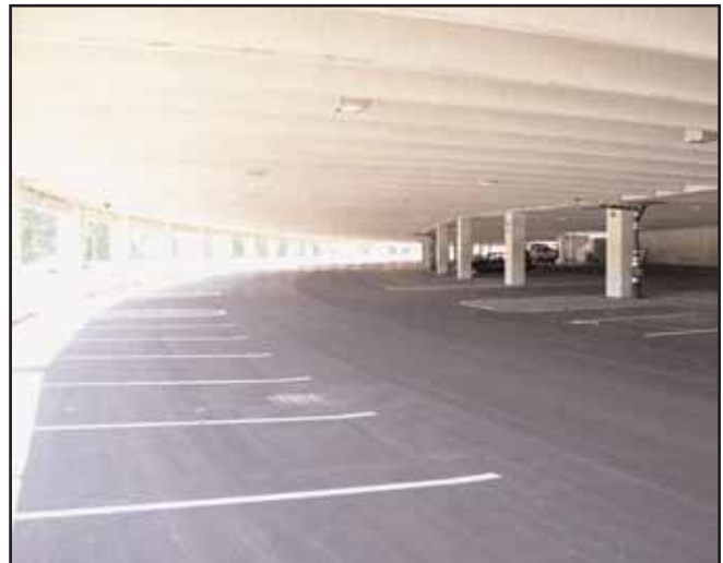
Inside of Liberty Mutual Corporate Campus Parking Garage
