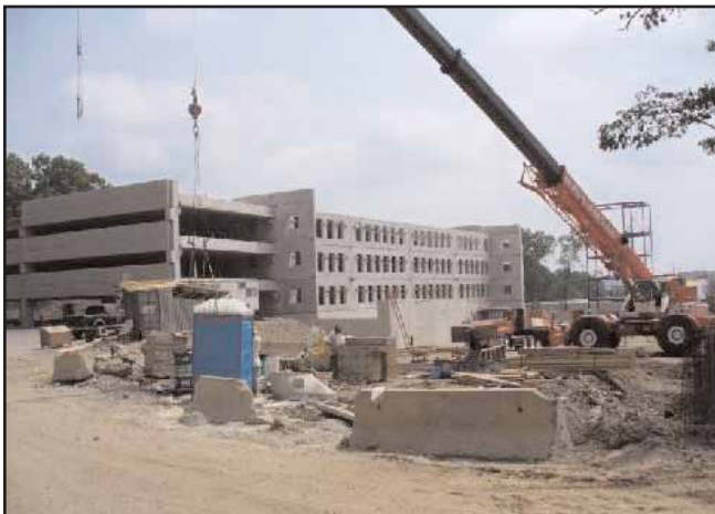
Construction of Reservoir Woods Parking Garage Photo by: C & A
