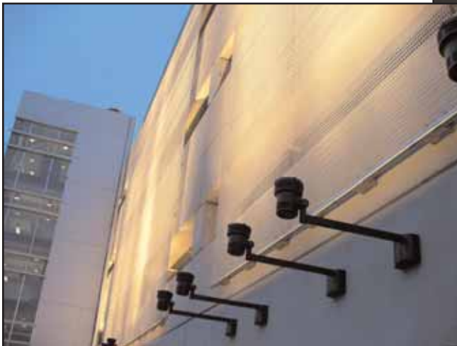
Screen and lighting attach directly to precast exterior Photo by: C & A
