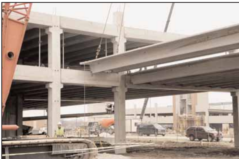
Precast parking structure being erected
