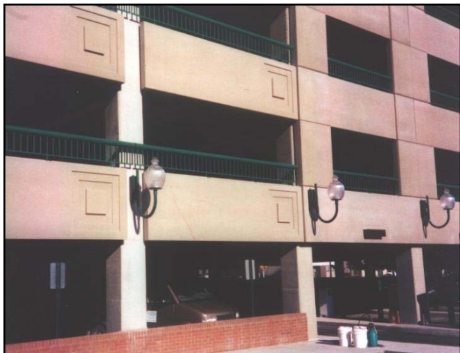
Simple details dress up simple spandrels for Jamestown garage.
