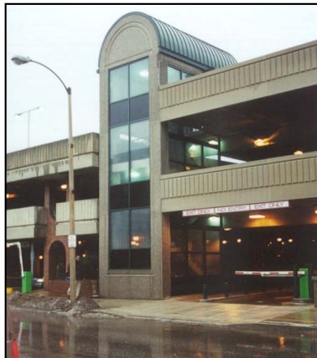
Precast panels add highlights.
