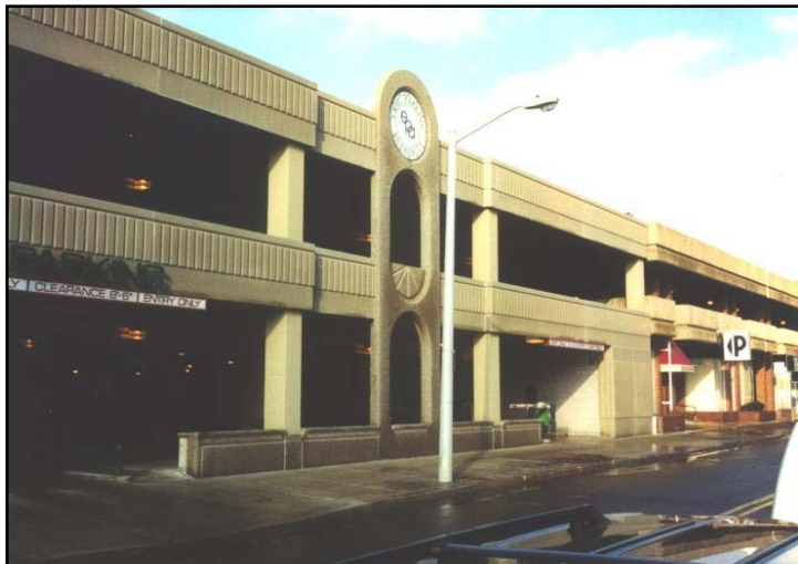
Precast to attract the customers.
