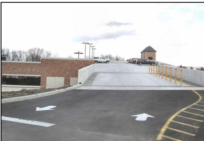
Bridge to roof top parking.
