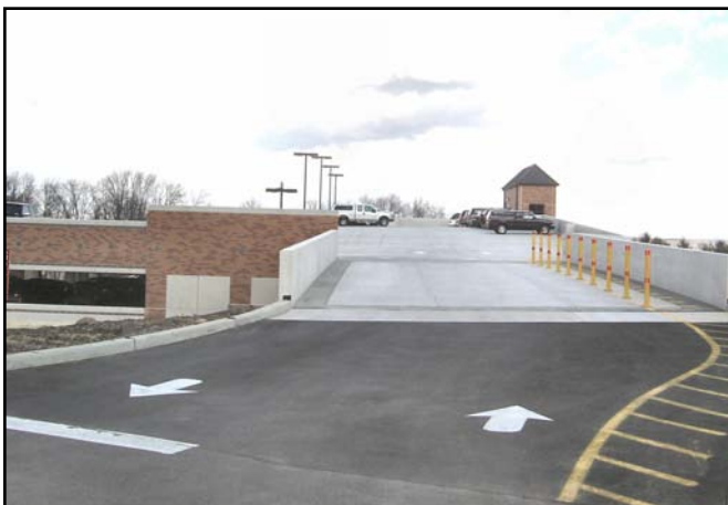
Bridge to roof top parking.
