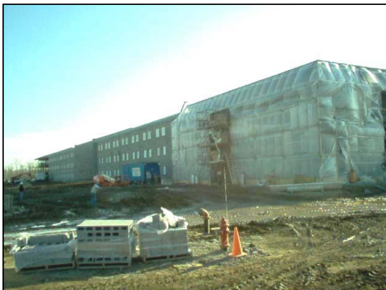
Tented project to allow winter construction of masonry
