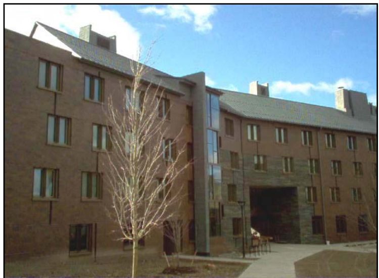
Dormitory complete; brick and stone added for campus compatibility Photo by Oldcastle Building Systems
