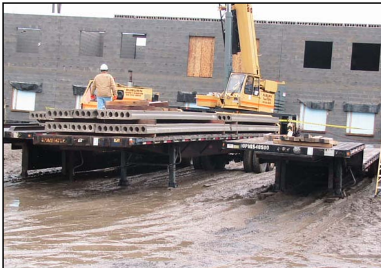
8" hollow core plank designed for blast loading
