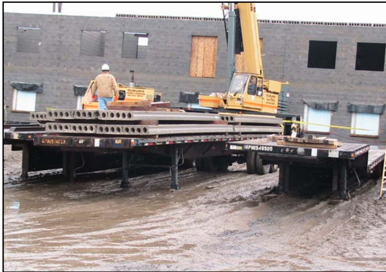
8" hollow core plank designed for blast loading
