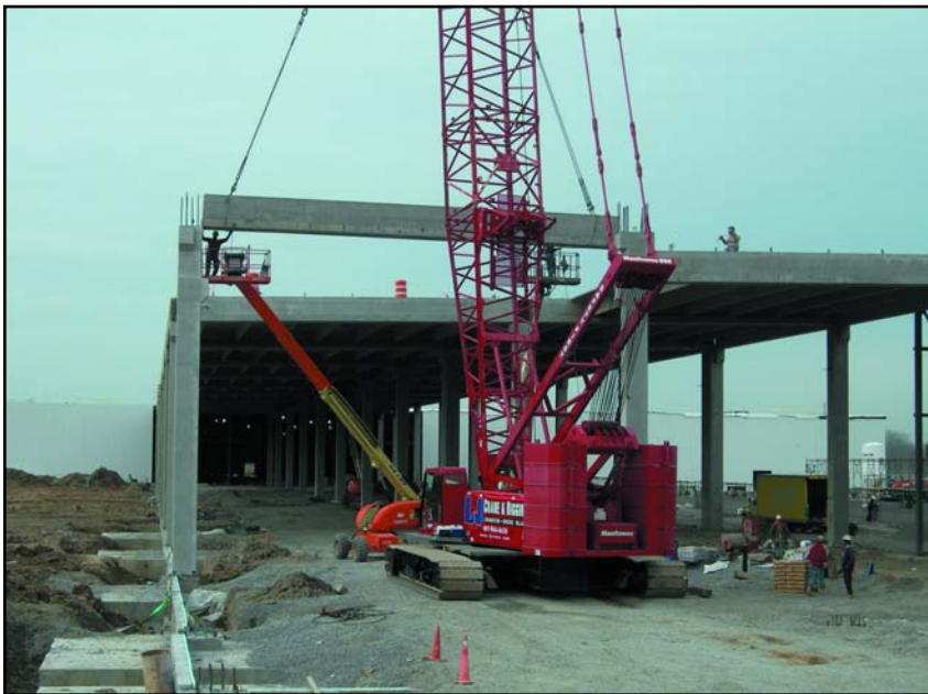
Moment resisting framed structure installation.
