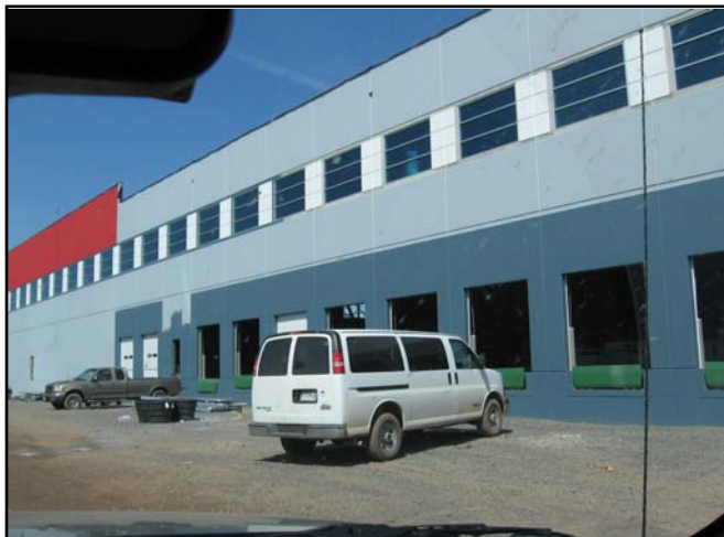
Loading dock openings cast into panels.
