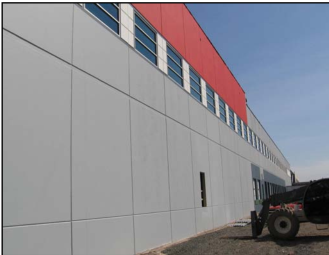
LEED - Clean site during construction.
