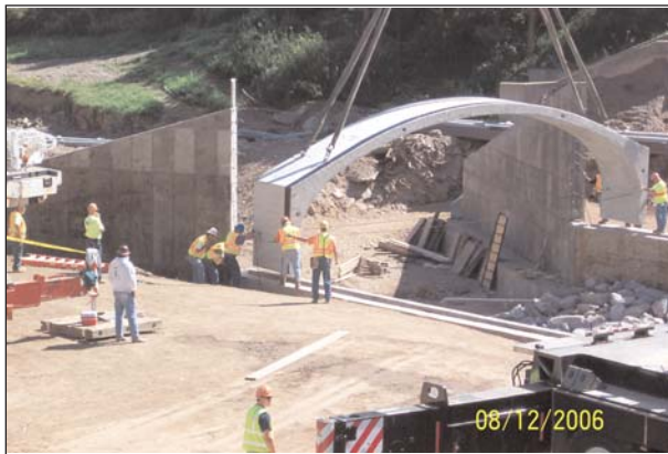
Installation of first ConSpan section.
