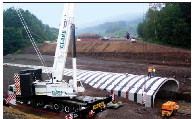
Installation of precast units was part of 24/7 emergency construction cycle.
