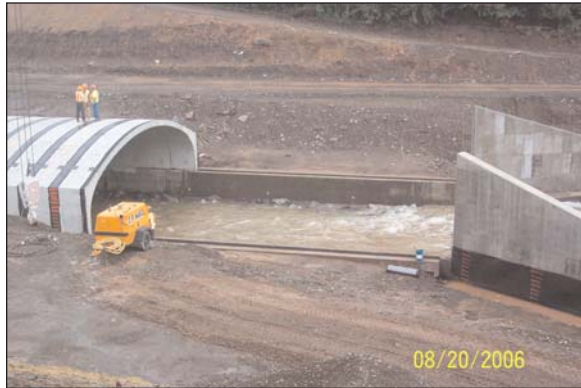
Installation over surging water.
