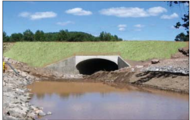
I-88 over Carrs Creek completed.
