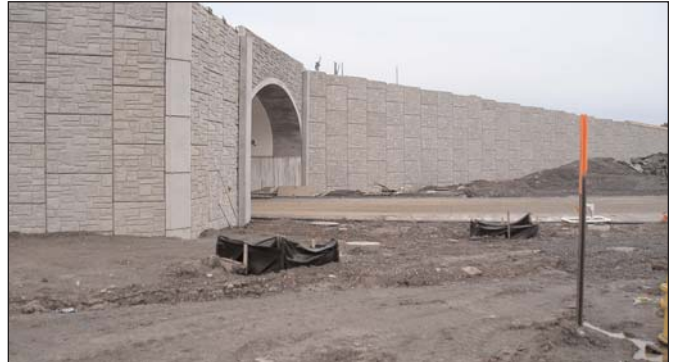
Installation of tunnel arch members
