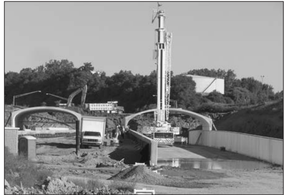
Installation of tunnel arch members
