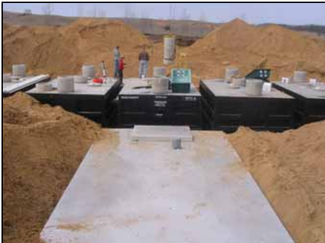
Setting top of 38,000 gallon Equalization Tank
