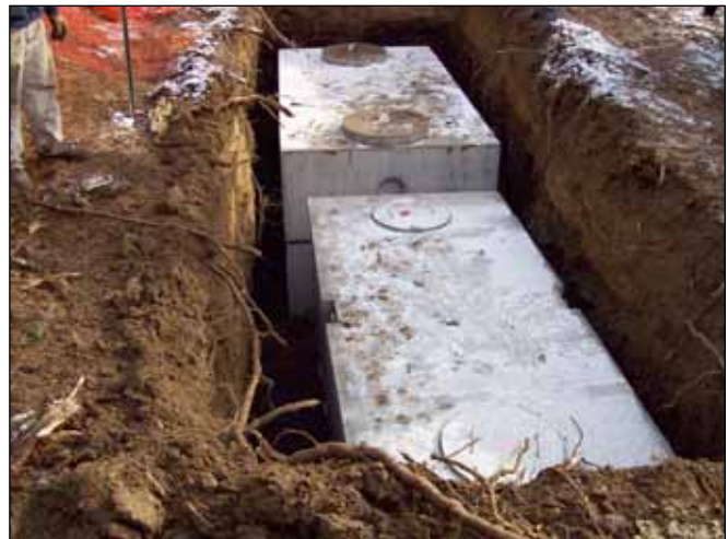
Septic tank (rear) and pump chamber just after setting
