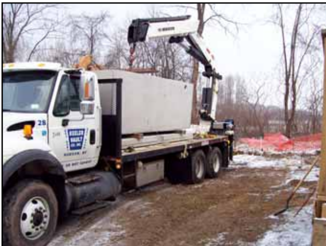
Pump chambers are set directly by the delivery truck
