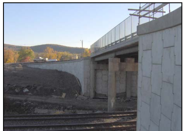
After Rehabilitation, using MSE panels
