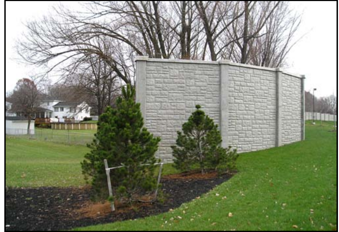
Attractive sound walls enhance neighborhood
