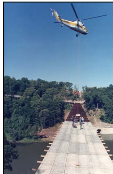
Helicopter setting replacement deck slabs
