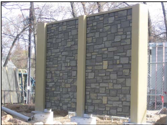
Community selected sound/security wall Photo by Hanson Pipe & Product
