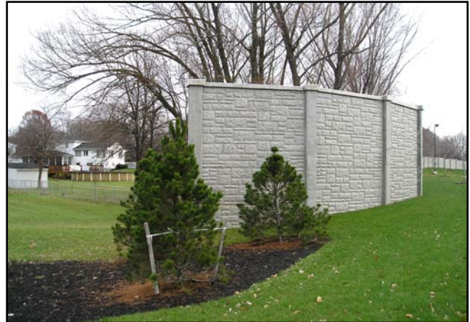
Attractive sound walls enhance neighborhood
