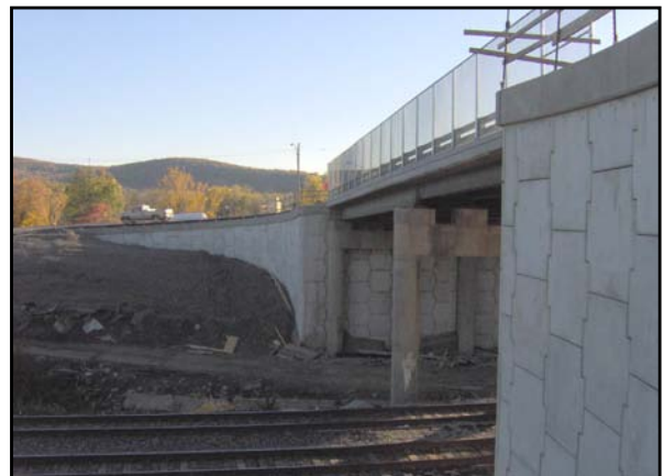
After Rehabilitation, using MSE panels
