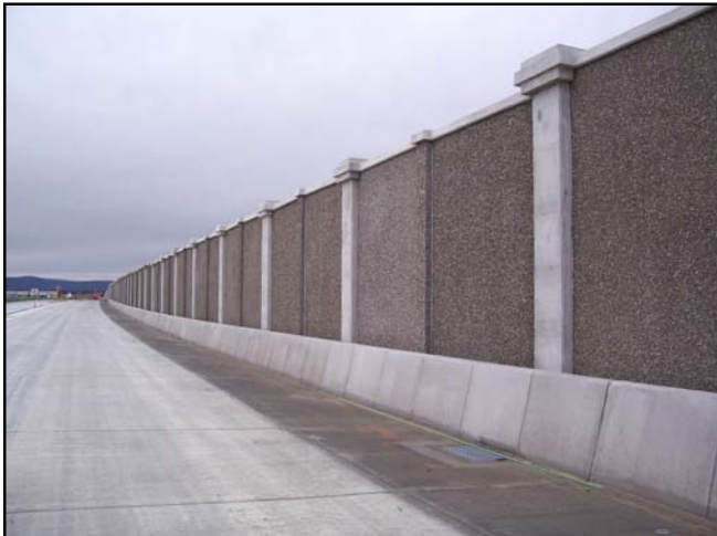
New Soundwall on I-86 Conversion, Horseheads, NY Photo by: Binghamton Precast
