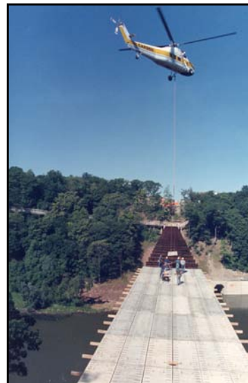
Helicopter setting replacement deck slabs
