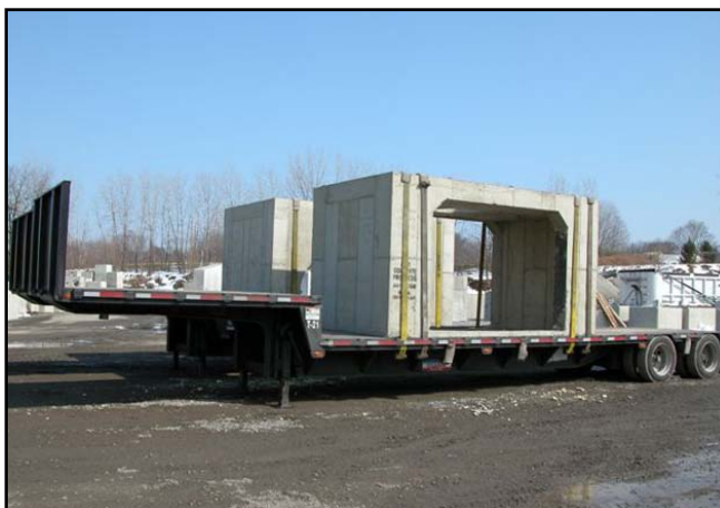
Meadowlands drainage structures, with diagonal corners to strengthen large openings
