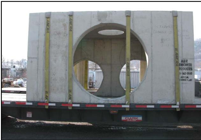
Meadowlands drainage structures, average weight 21 tons, with openings
