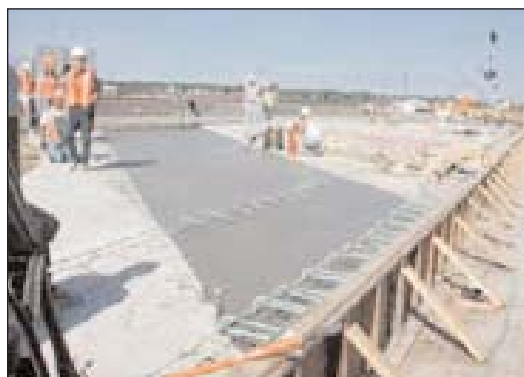
Hand finishing of ECC link slab on Grove Street Bridge project.
