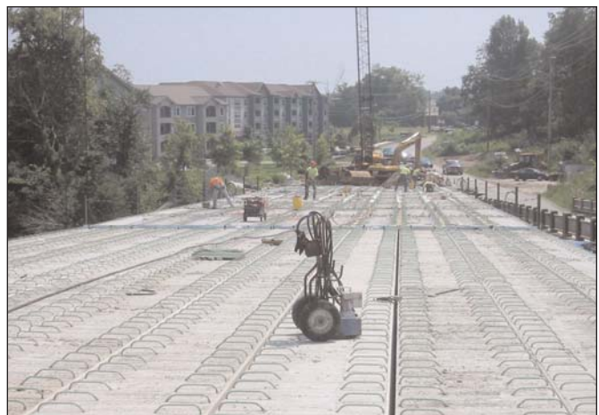
Concrete Greenfield – epoxy coated composite bars await deck pour.
