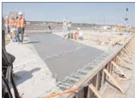
Hand finishing of ECC link slab on Grove Street Bridge project.
