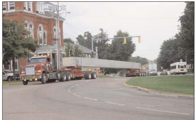
Transporting 103.5' beams over small town roads.
