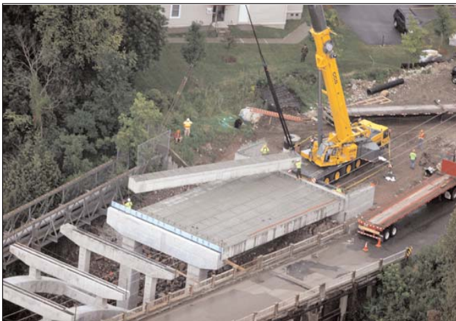
Simple installation of 60 foot long box beams.
