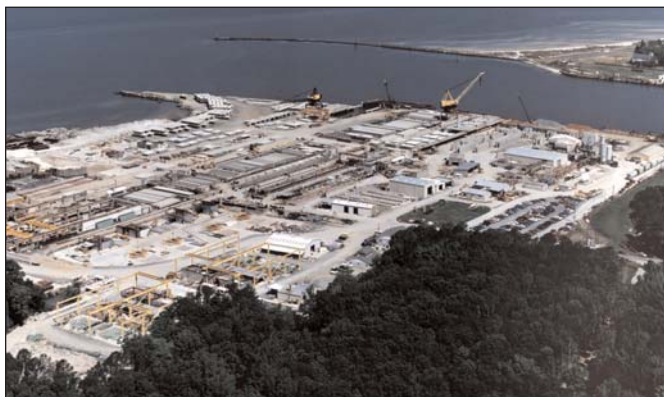
Bayshore Concrete Products, Cape Charles Plant. Photo by Bayshore Concrete Products.
