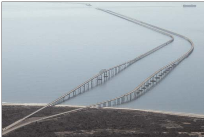
17 Mile Long Chesapeake Bay Bridge Tunnel. Photo by Bayshore Concrete Products.
