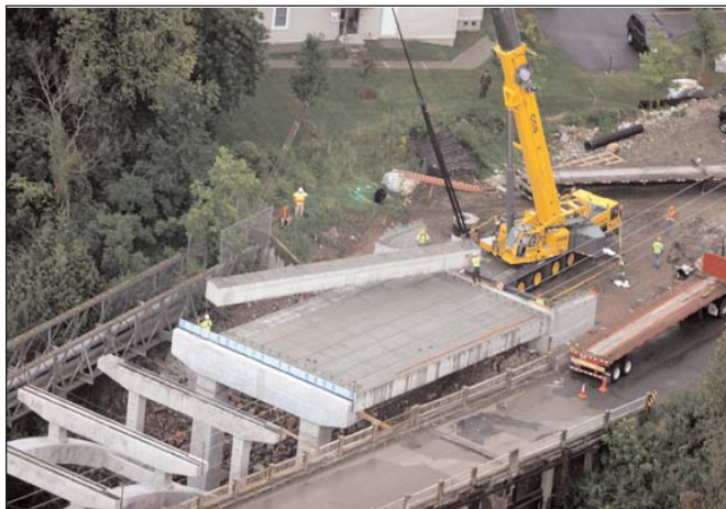
Simple installation of 60 foot long box beams.
