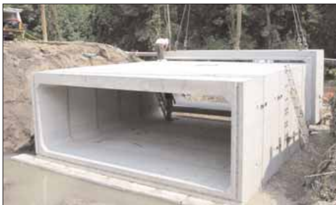
Swinging last unit smoothly into place Photos by Kistner Concrete Products
