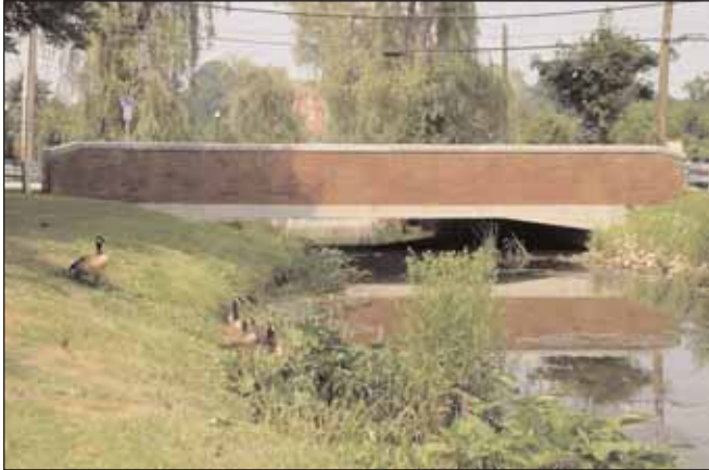
New "old" bridge in downtown Mt Kisco, NY Photos by The Fort Miller Co.
