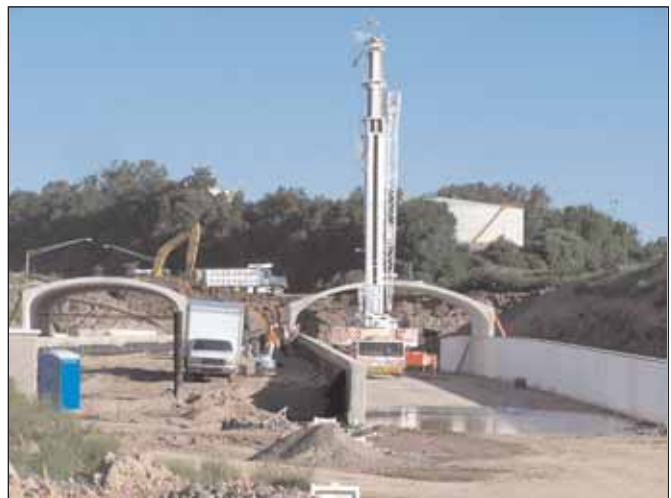
Installation of tunnel arch members
