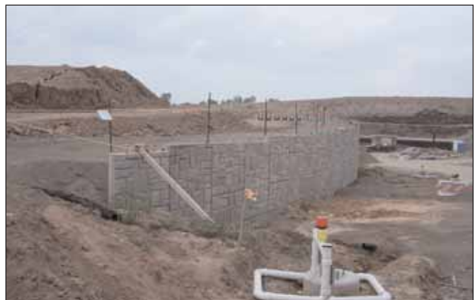
Stone faced precast concrete retaining walls
