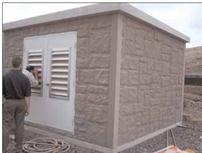
Stone faced precast concrete utility building
