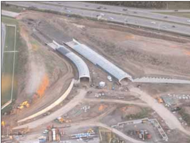
Pilot's view of project site
