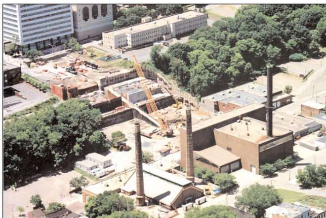
Stepped site preparation.
