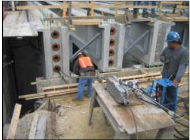
Running Post-Tensioning Strands into Ducts
