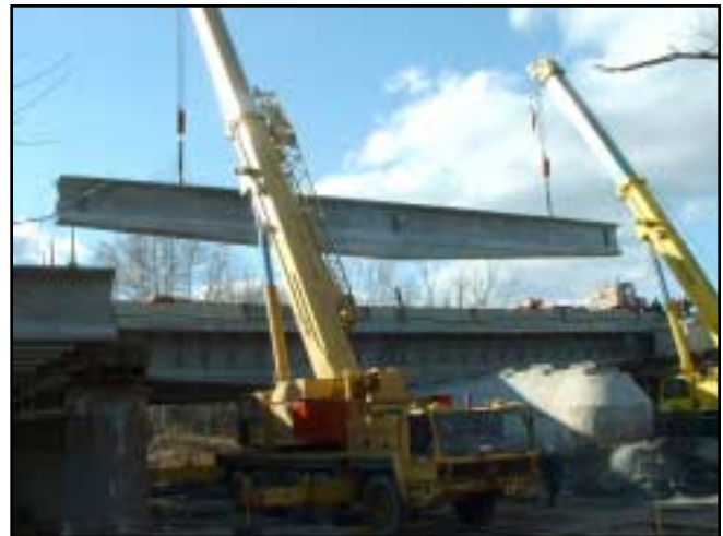
Installation of Tapered Center Segment Beams
