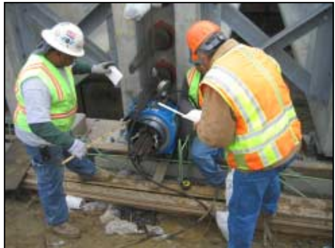
Gang Stressing Strands in P/T Ducts
