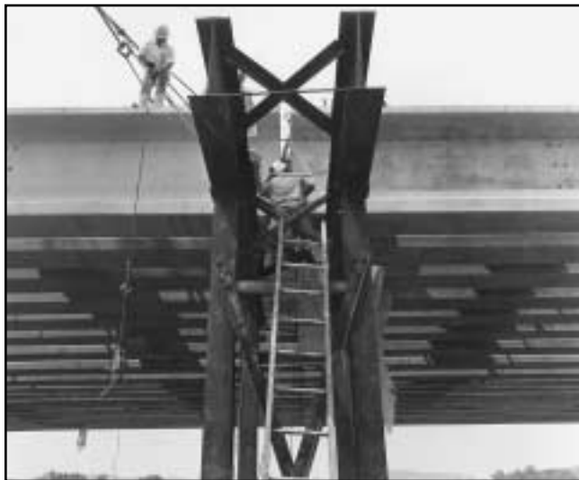
Figure 2. Girder splice
