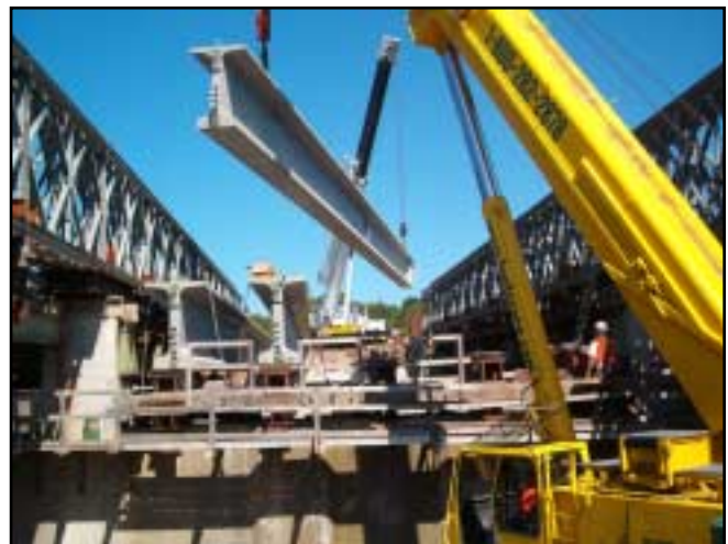
Installing 128-8" Modified NEBT Girders on Temporary Supports in Foreground
