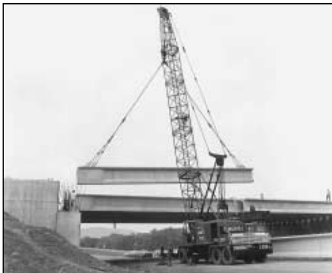
Figure 1. Erection of girder segment
