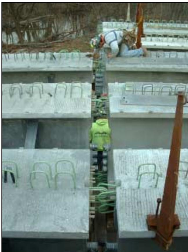
Abutting Beams Ready for Closure Pour Work
