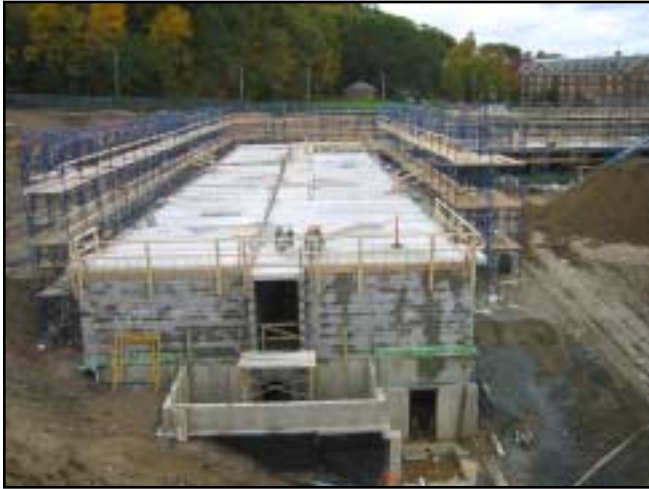
Construction underway for new student apartment complexes Photos by J. P. Carrara & Sons
