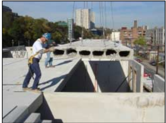
Installation of load bearing interior walls, elevator shaft walls, and hollow core plank proceeds quickly
