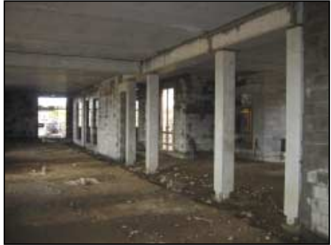
Precast beams, columns and lintels enable first level open areas
