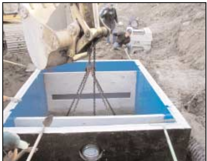
Custom Oil & Grit Separator for Stormwater Flow
