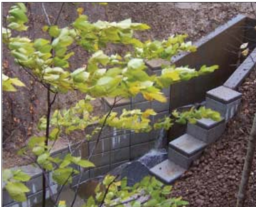
Culvert wall using modular stay in place block.
