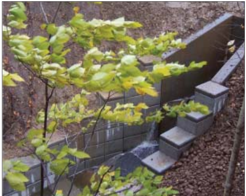
Culvert wall using modular stay in place block.
