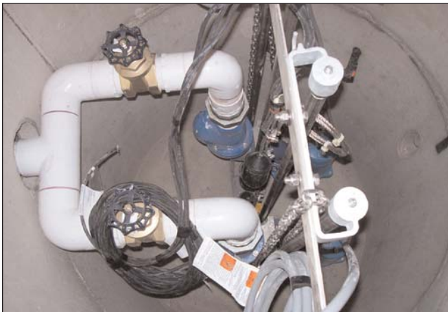
Wet well ready to ship.
