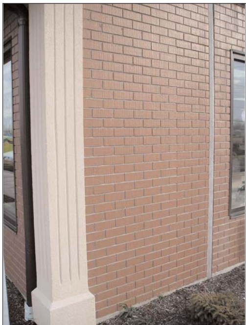
Brick face precast concrete panel.
