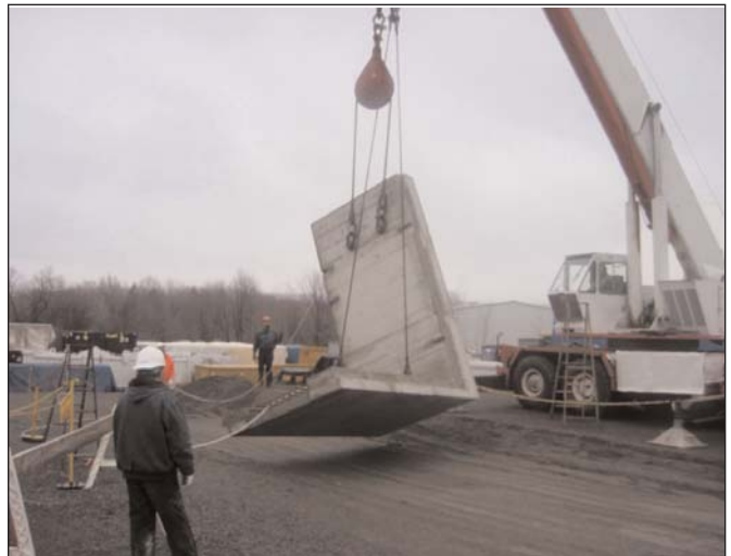
Positioning wall/half floor segment.
