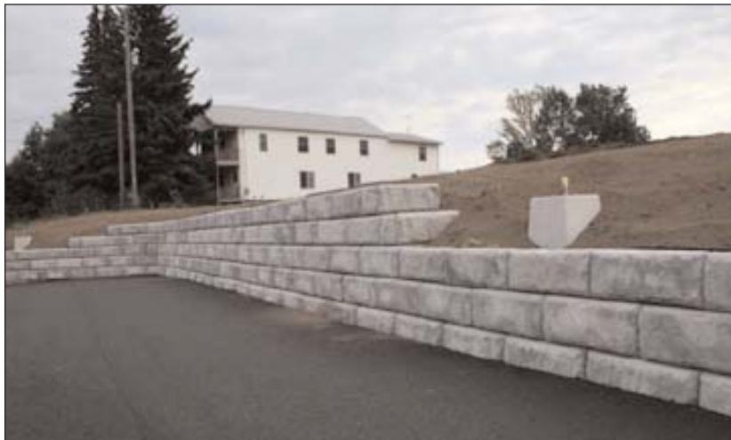
Redy Rock retaining wall, West Seneca Bus Garage.
