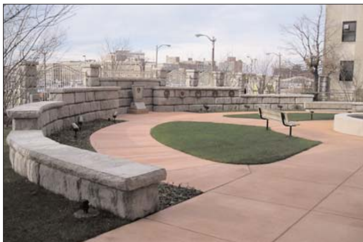
Precast blocks form courtyard surround.
