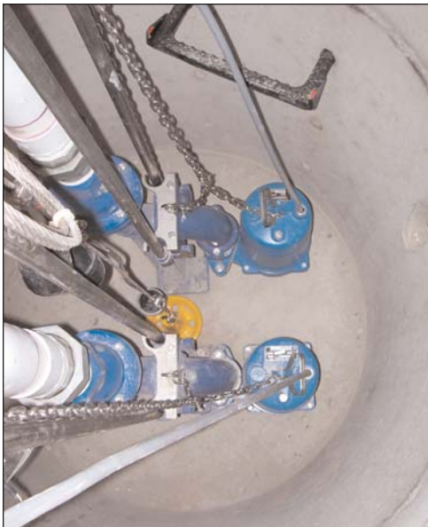
Preparing preassembled wet well.
