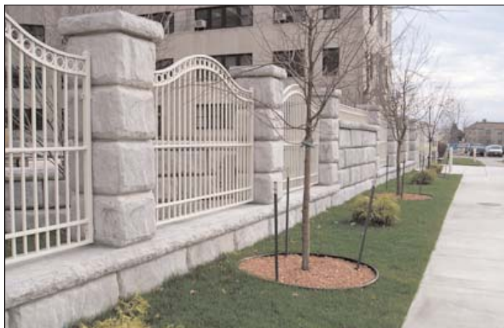
Precast blocks bolster iron fence.
