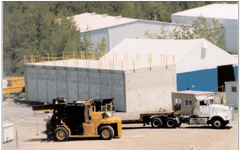
Each structure was erected in 1 day.
