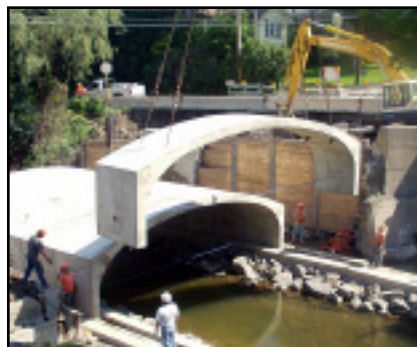
Con-Span arch units quickly, easily installed.
