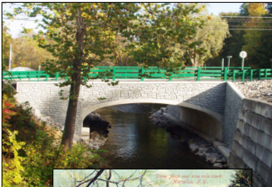
Con-Span arch units quickly, easily installed.
