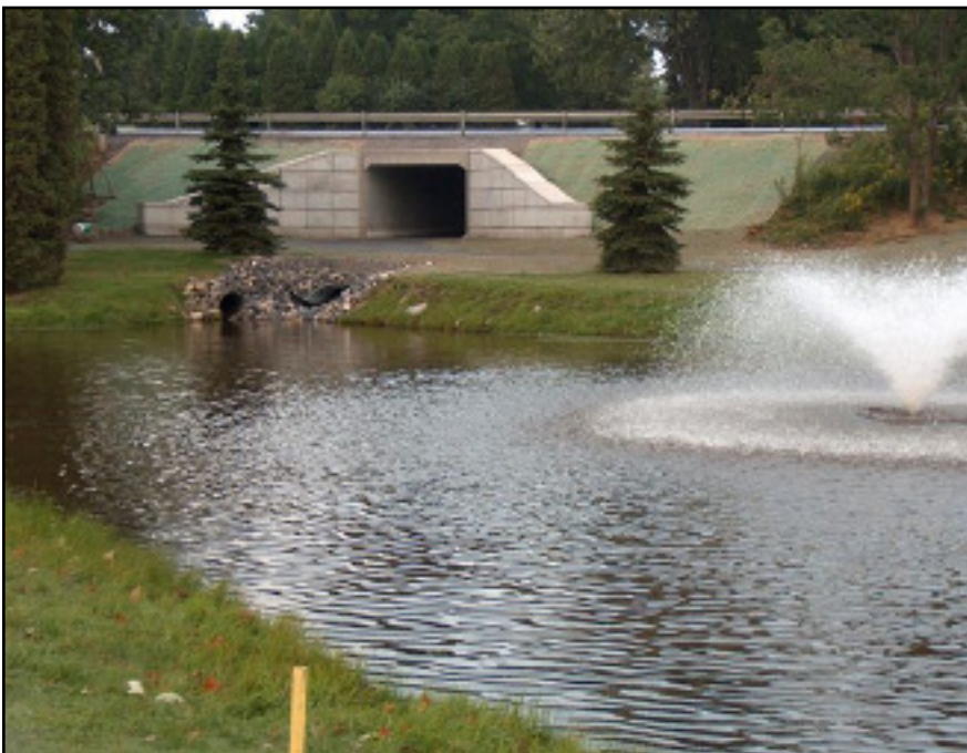
Photos by Kistner Concrete Products.
