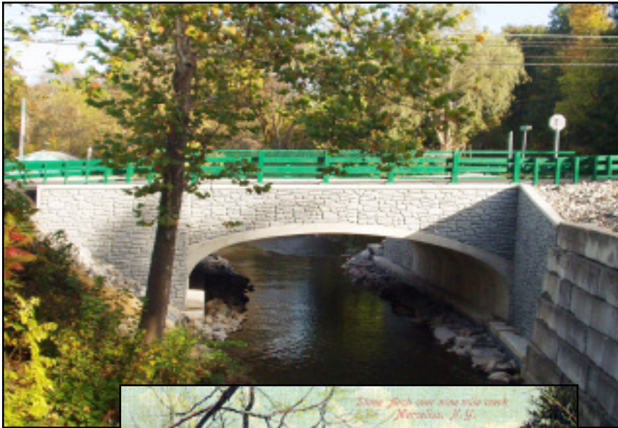
Con-Span arch units quickly, easily installed.
