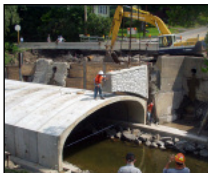
All precast components supplied by Kistner Concrete Products, Lockport plant.
