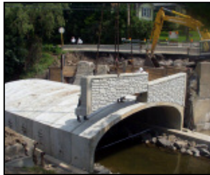
Stone faced precast walls plant cast with form liners.
