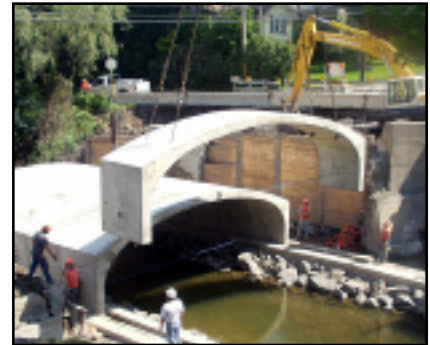
Con-Span arch units quickly, easily installed.
