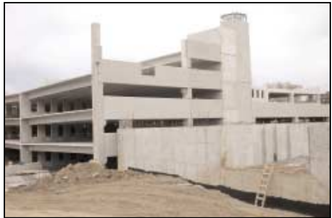
Garage tight against theater retaining wall Photos by Unistress Corp
