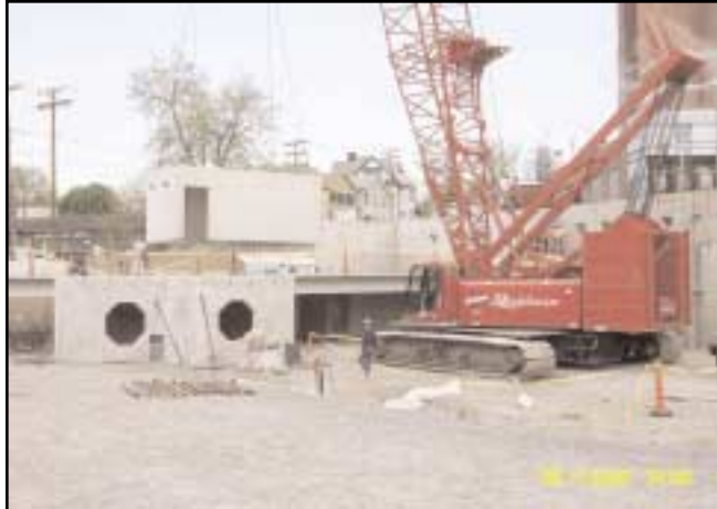
Columbia - Stair box unit hoisted into position
