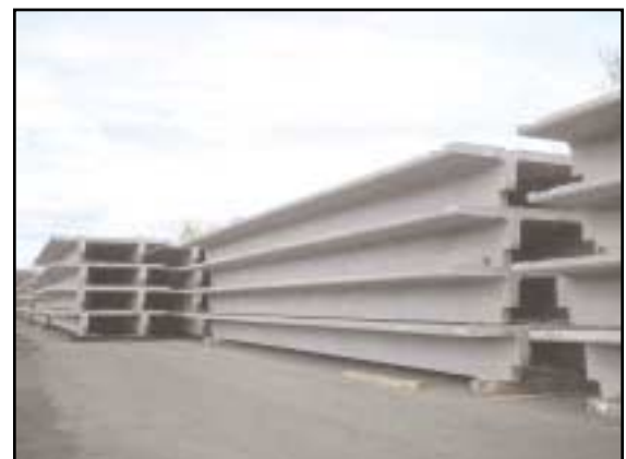
15' wide pretopped tees stretch out for half a mile prior to erection (photos by L.C. Whitford)
