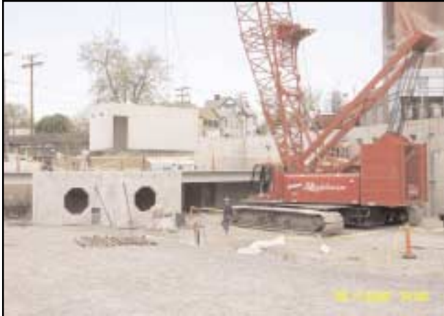
Columbia - Stair box unit hoisted into position
