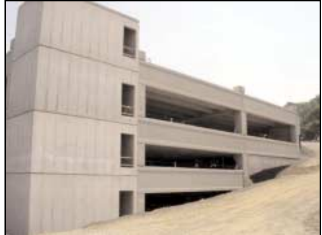
Columbia - Finished stair tower and garage nearing completion
