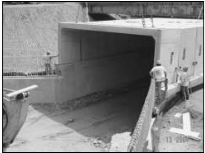
Photos by Riefler Concrete
