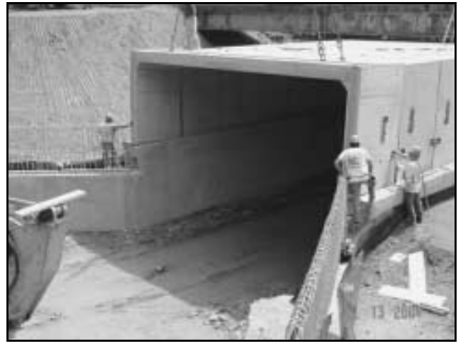
Photos by Riefler Concrete
