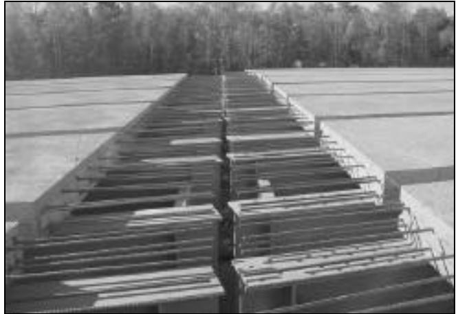
Steel splice plates and connecting diaphragms were pre-drilled at this time to minimize jobsite time.
