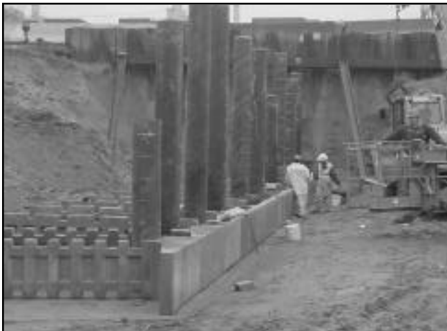
The units were placed around the pipe piles that supported the concrete abutment cap beams
