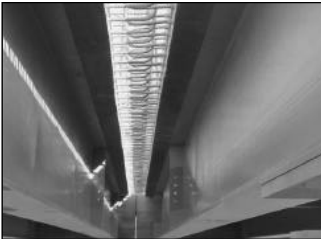
Steel splice plates and connecting diaphragms were pre-drilled at this time to minimize jobsite time.
