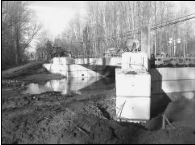
Blocks cast with stone facing
