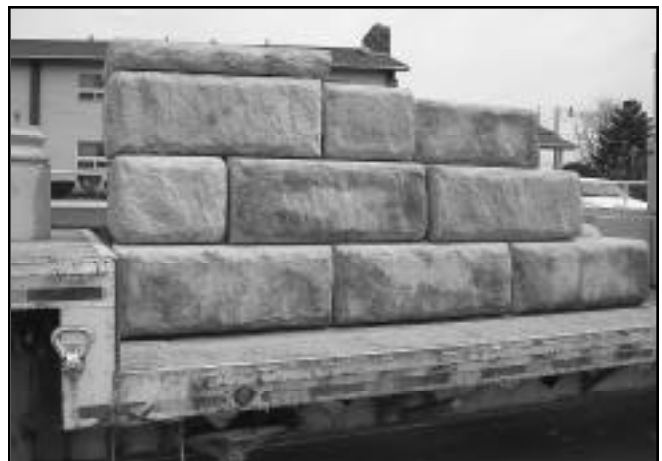
Precast block element abutment support prestressed box beam bridge units
