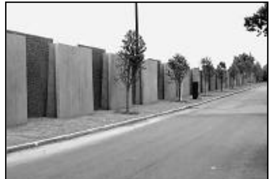
A finished sound barrier separates the local homes from the busy express lanes beyond
