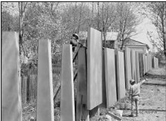
I-490 Gateway Sound Barrier Installation
