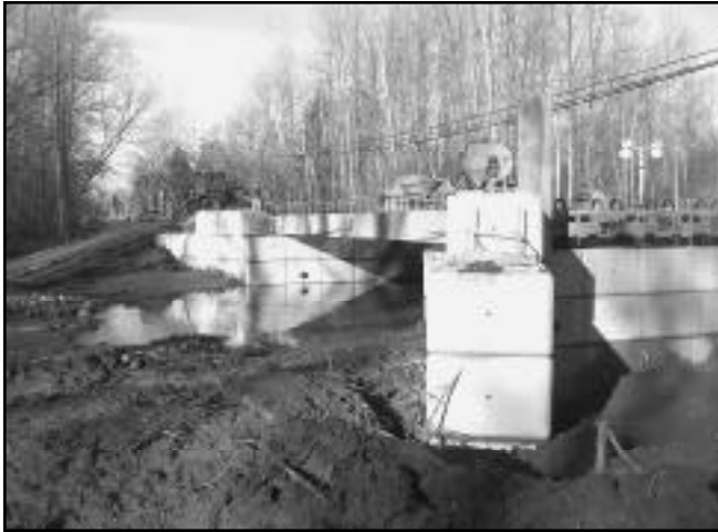
Blocks cast with stone facing
