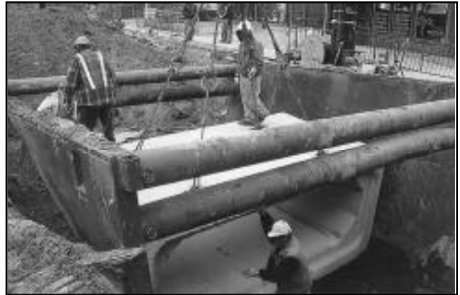
Precast aids speedy completion in a tight site
