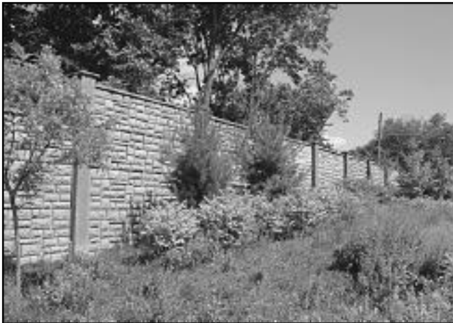
Hutchinson River Parkway, Rye Brook, NY
