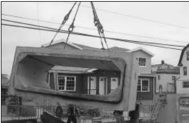
Rubber gasket pre-applied to the box culvert tongue
