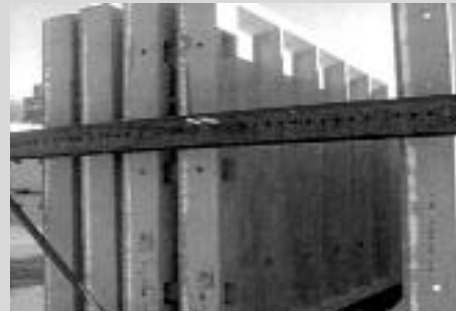
Insulated CarbonCast foundation panels impervious to moisture
