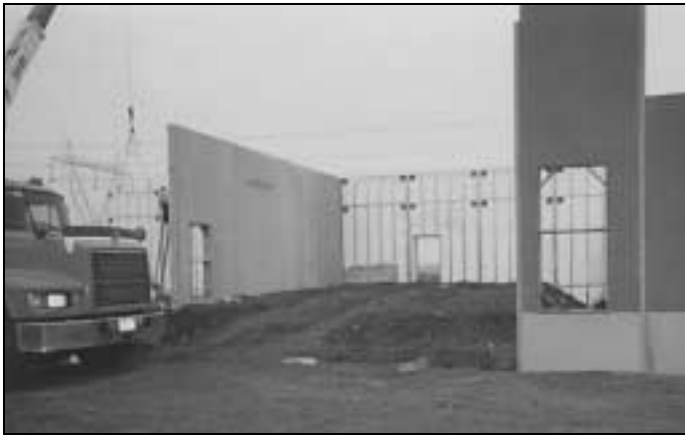
Brick, brushed, and insulated surfaces
