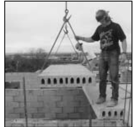
Curry College 8' Plank Erection
