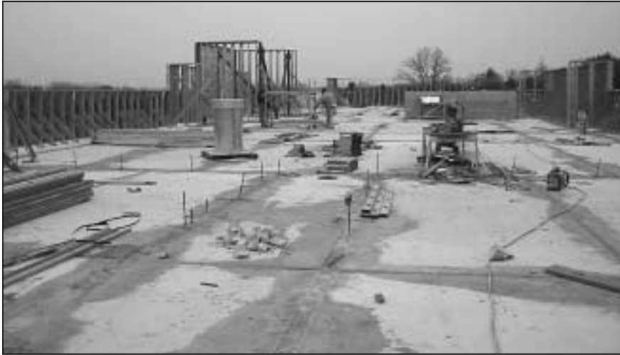
Plank deck provides safe work deck for following trades
