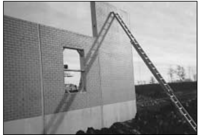
Brick wall panel with window opening
