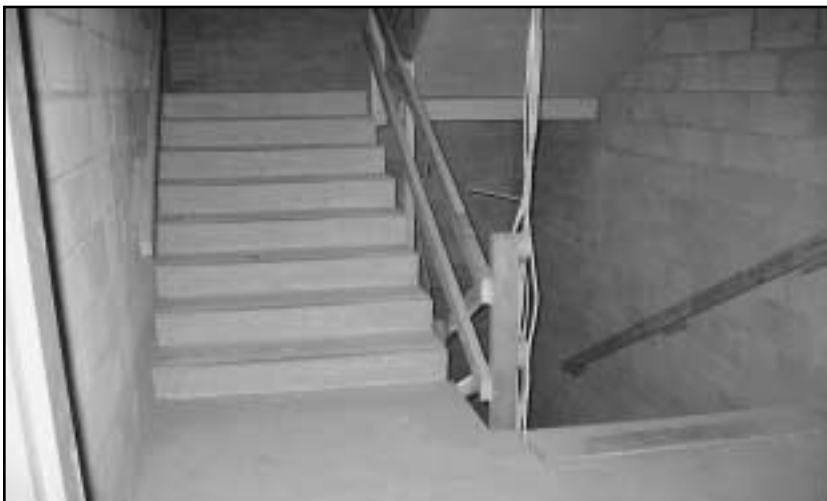
Precast concrete stairs and landings
