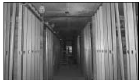
Clean ceiling lines down corridor facilitates mechanical work
