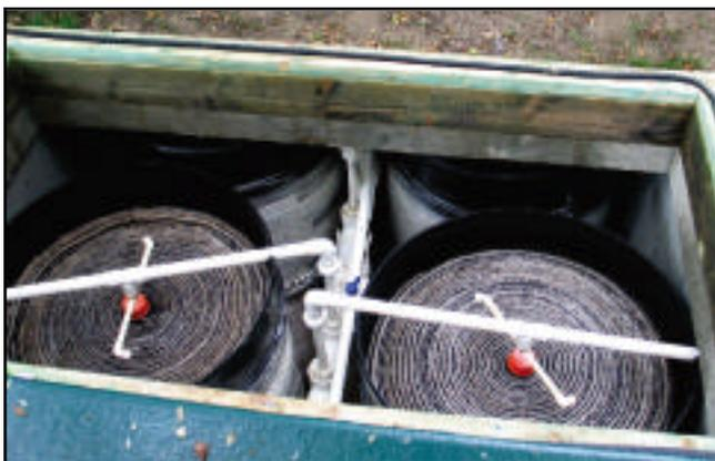
Coils of textile and peat receive aerobic effluent from the septic tank, which is re-circulated via a timed system
