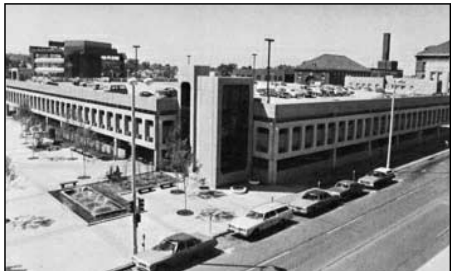
Rock Island Parking Structure
