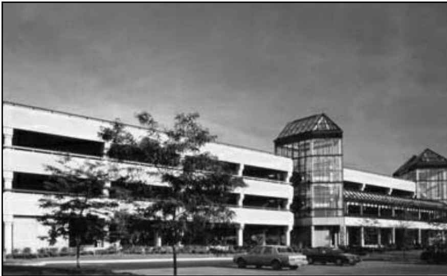
Blue Cross-Blue Shield Parking Structure
