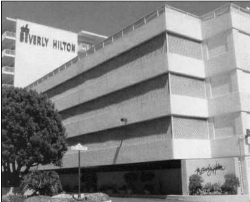
Beverly Hills Hilton Parking Structure
