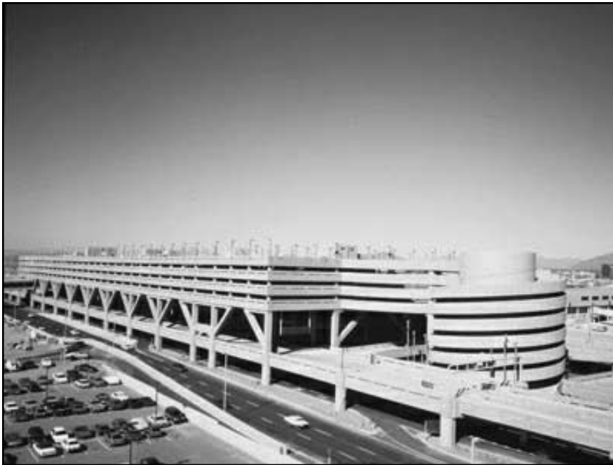
Sky Harbor International Airport
