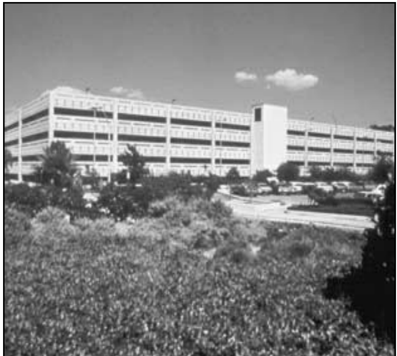
Baylor Hospital Parking Structure
