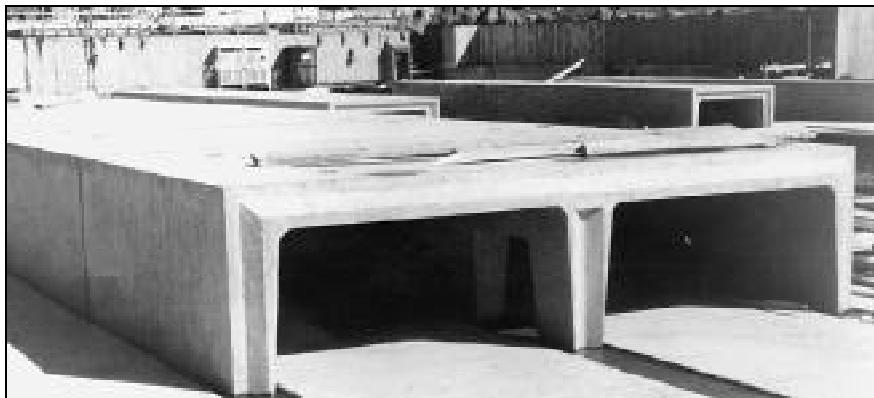
Precast ducts are shown for storage of CSOs in New York City. photo from Precast Solutions
